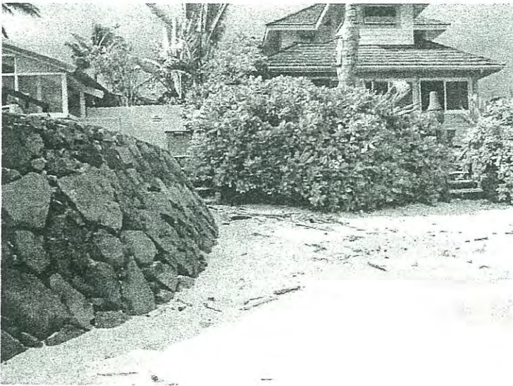
View of Parcel 11 seaward frontage. Seawall is hidden by naupaka vegetation. Curved seawall on left fronts Parcel 10.
