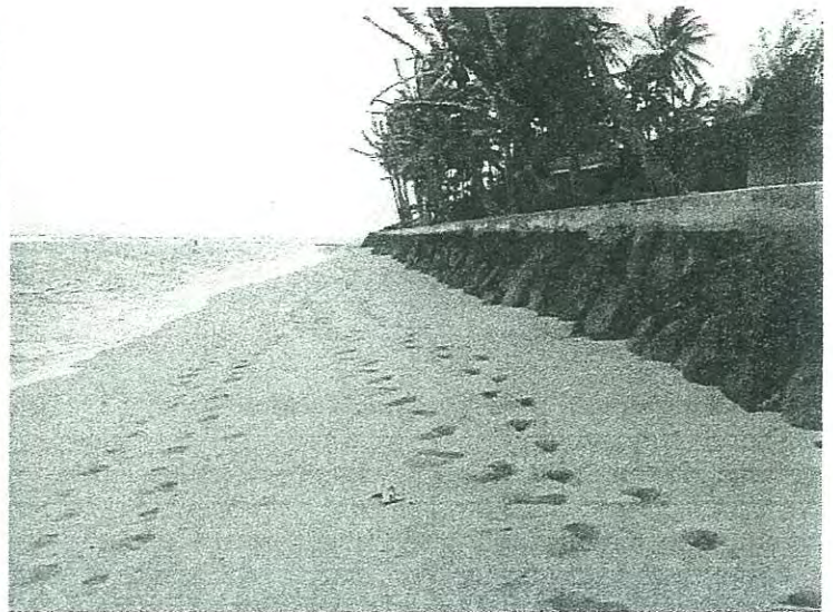
View eastward along the beach fronting the Mokuleia Beach Colony seawall. Note the narrow and steep beach profile.
