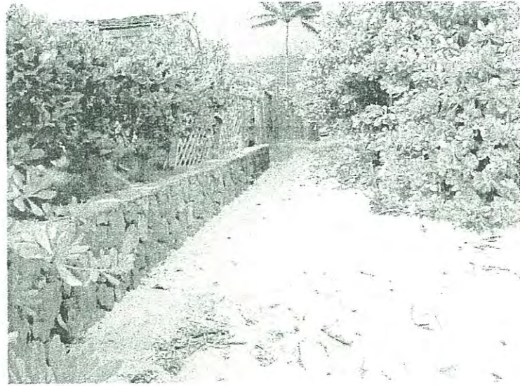
View mauka along private right-of-way. The CRM wall on left is Parcel 11's return wall.
