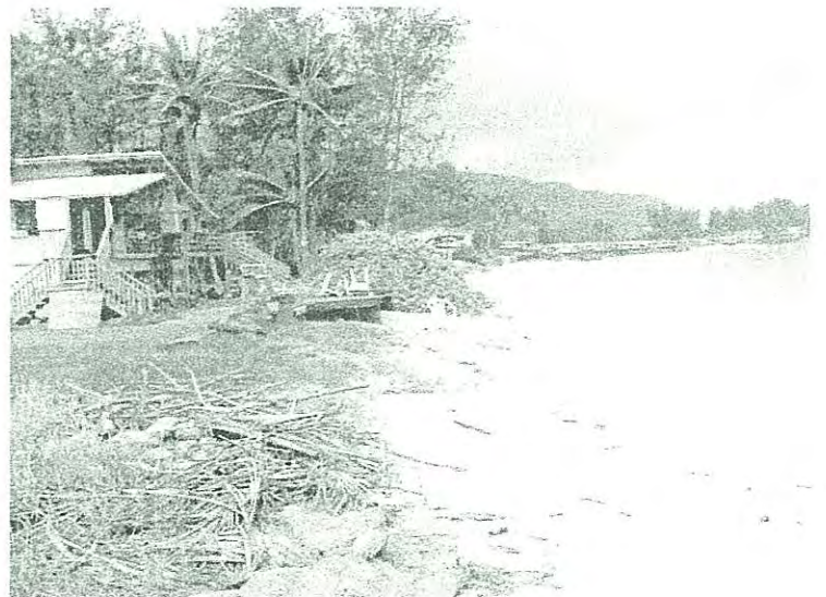
Shoreline fronting Parcel 20 on east side of stream. Note debris line at edge of vegetation.
