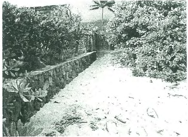
View mauka along private right-of-way. The CRM wall on left is Parcel 11's return wall.
