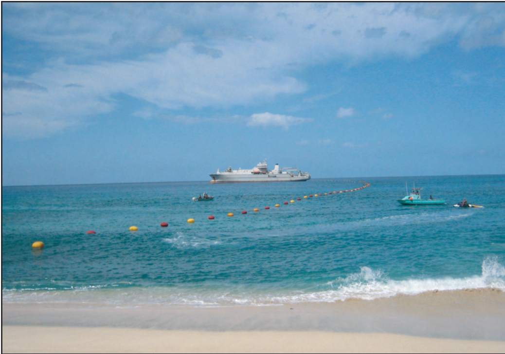
Cable with Floats Deployed from Cable Ship
