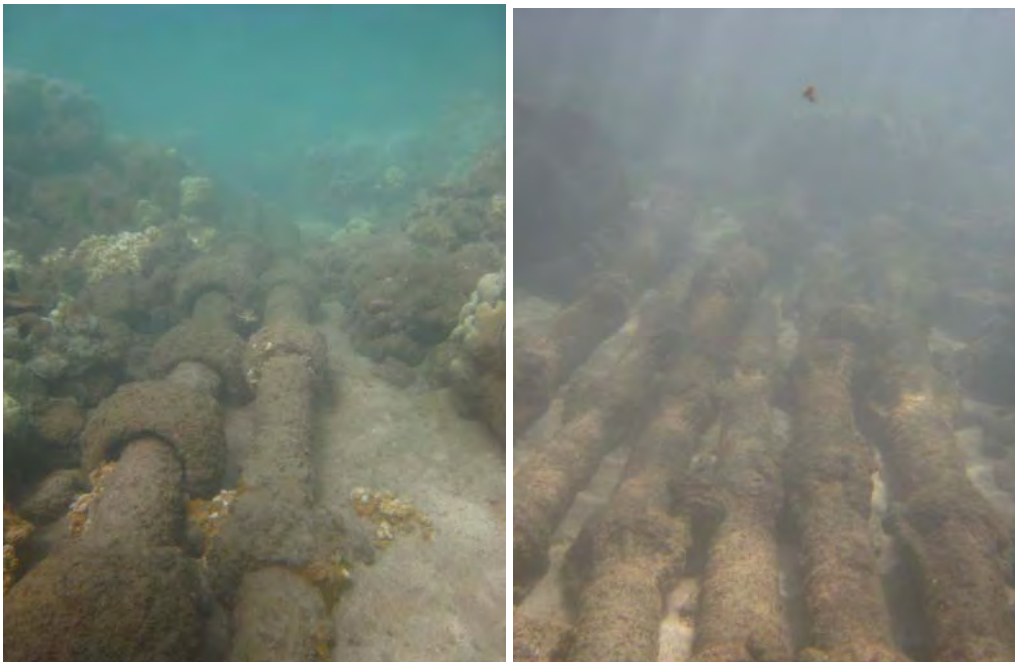
GTE (left) and PLNI (right) Cables in Articulated Pipe, at 1 m Water Depth
