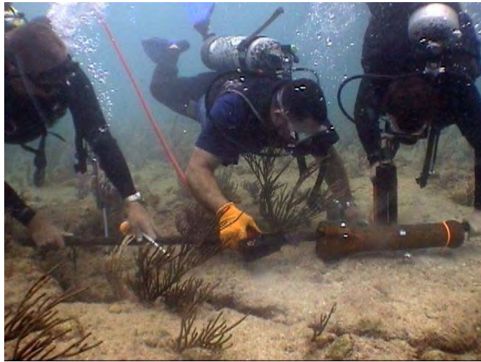
Stainless steel saddle clamps installed by divers.
