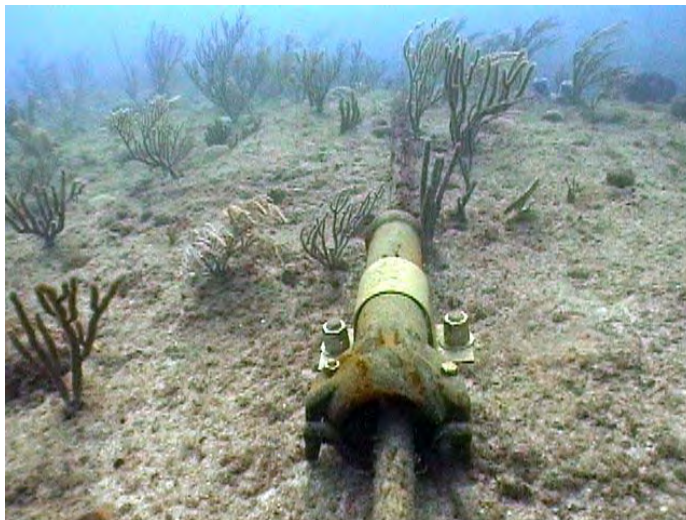
Saddle clamps secure cable to rock to prevent movement and scour.
