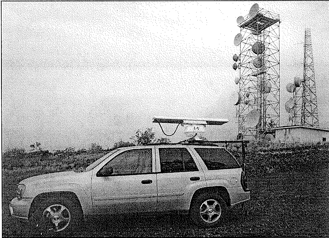
Figure 4. Topography, vegetation, and existing HELCO towers at the proposed 'Ānuenue radio relay tower site, Ka'ūpūlehu, Hawai'i.
