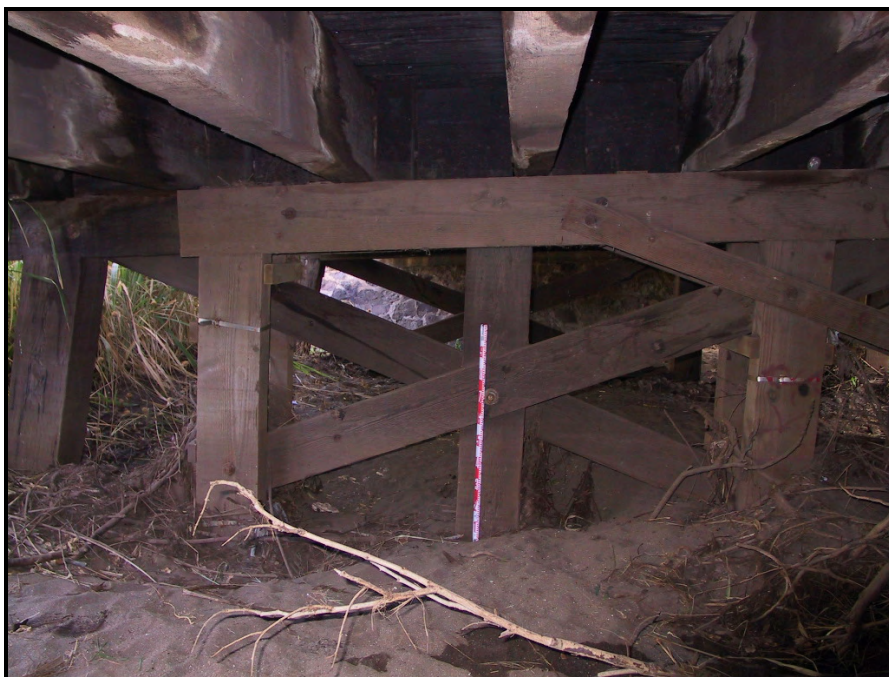
Figure 26. Photograph of SIHP # 50-80-07-6822, showing massive wooden beams, bents, and columns, and plank X-bracing, view to northwest/north
