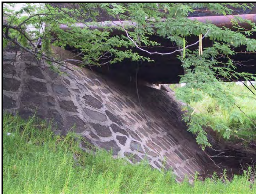
Figure 36. Photograph of SHIP # 50-80-07-6823, blue rock and mortar abutment, view to the west
