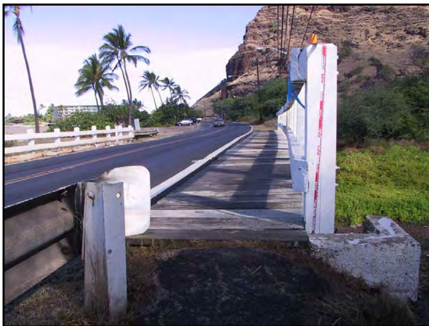
Figure 37. Photograph of SHIP # 50-80-07-6823, concrete corner reinforcement, wooden sidewalk and guardrail, view to northwest
