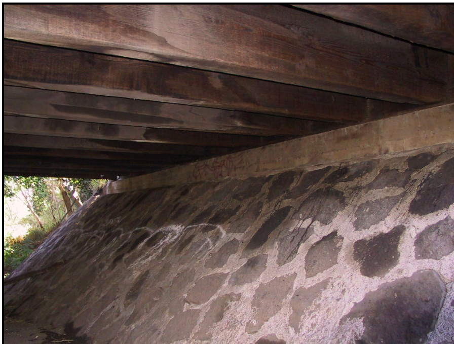
Figure 27. Photograph of SIHP # 50-80-07-6822, blue rock and mortar abutments, wooden beams and concrete end bent, view to north
