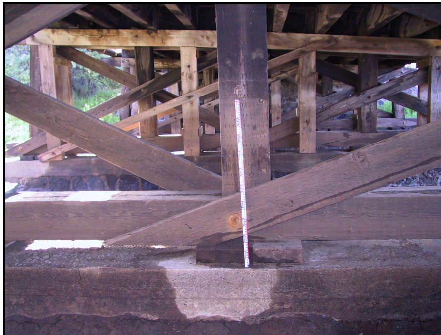
Figure 35. Photograph of SHIP # 50-80-07-6823 substructure, showing wooden columns, beams, planks, X-bracing, and the concrete and blue rock and mortar piers, view to south
