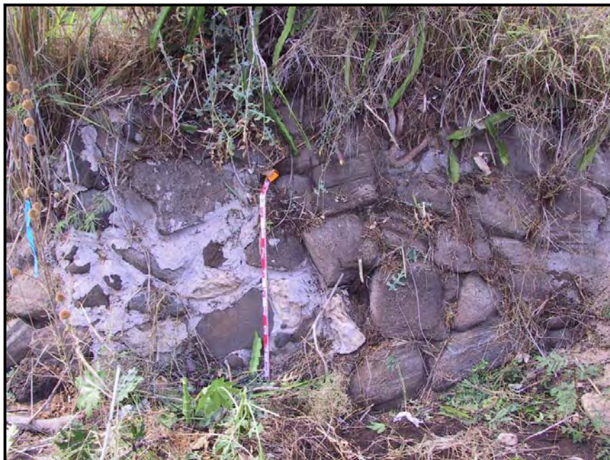
Figure 46. Photograph of the southern abutment of Feature B, SIHP # 50-80-12-9714, shot south, showing crude basalt boulder and mortar construction.
