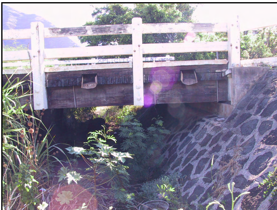
Figure 28. Photograph of SIHP # 50-80-07-6822, blue rock and mortar abutments with concrete reinforcement at corners, view to north
