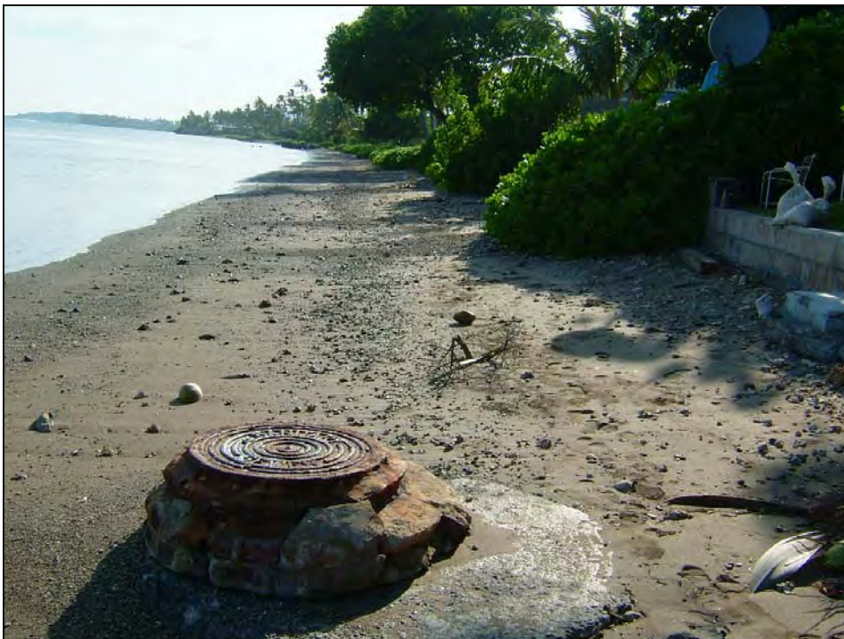
Figure 32. Segment 1 sewer line located along Wailupe Beach, view to the west. Manhole frame and cover to be replaced
