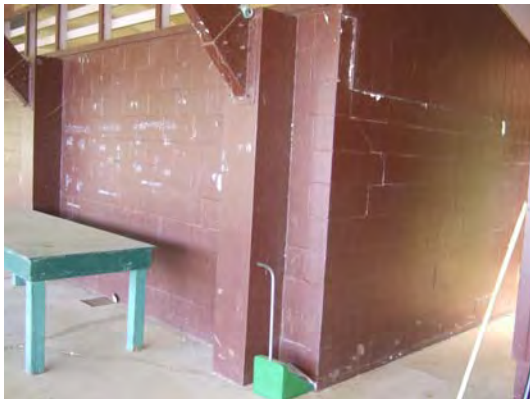
Damage to restroom wall – south wall
