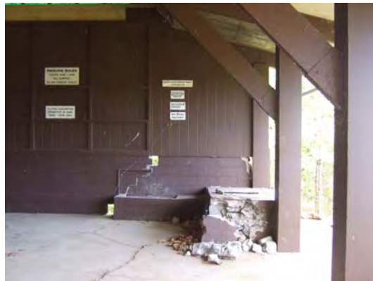
Damage to west wall – to be removed
