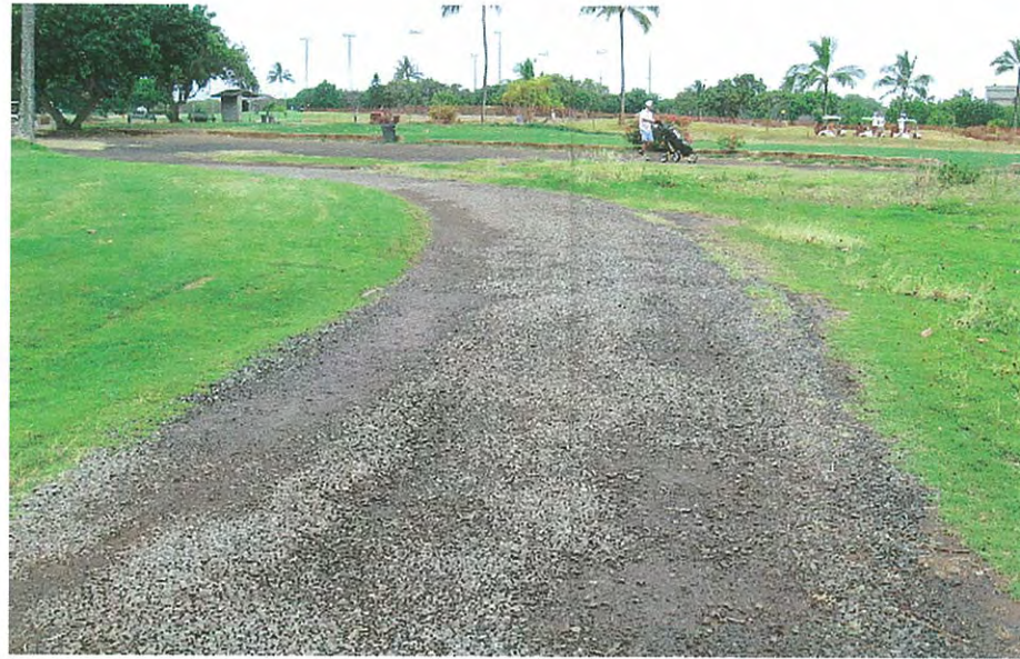
Photograph 2. Cart Path to 2nd Tee Box.
