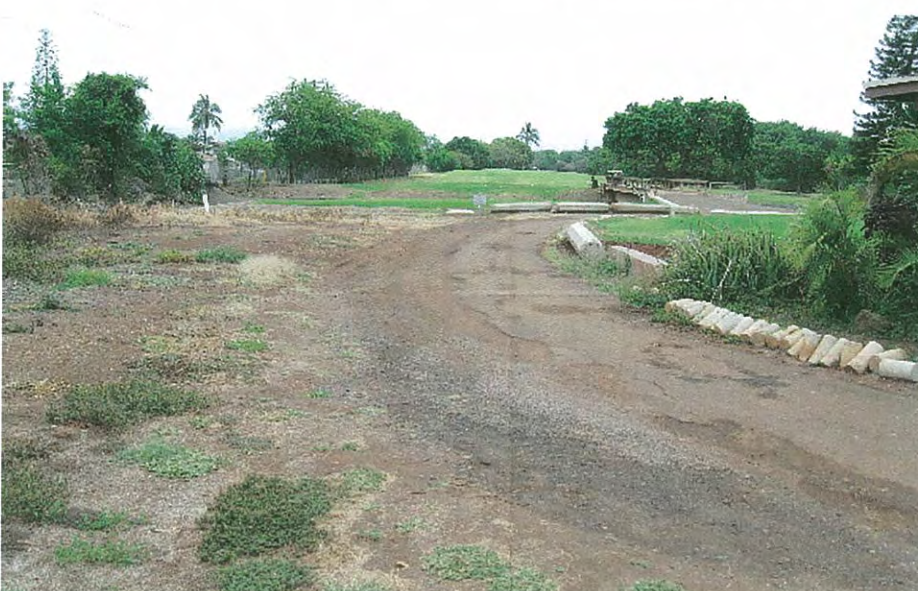
Photograph 6. Cart Path Behind the Comfort Station Near the 14th Tee.
