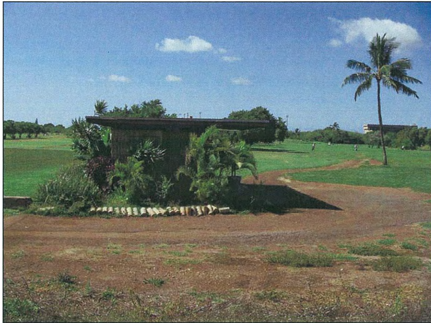
Figure 28. Photograph of restroom facility situated atop LCAs within the northwestern corner of the project area.
