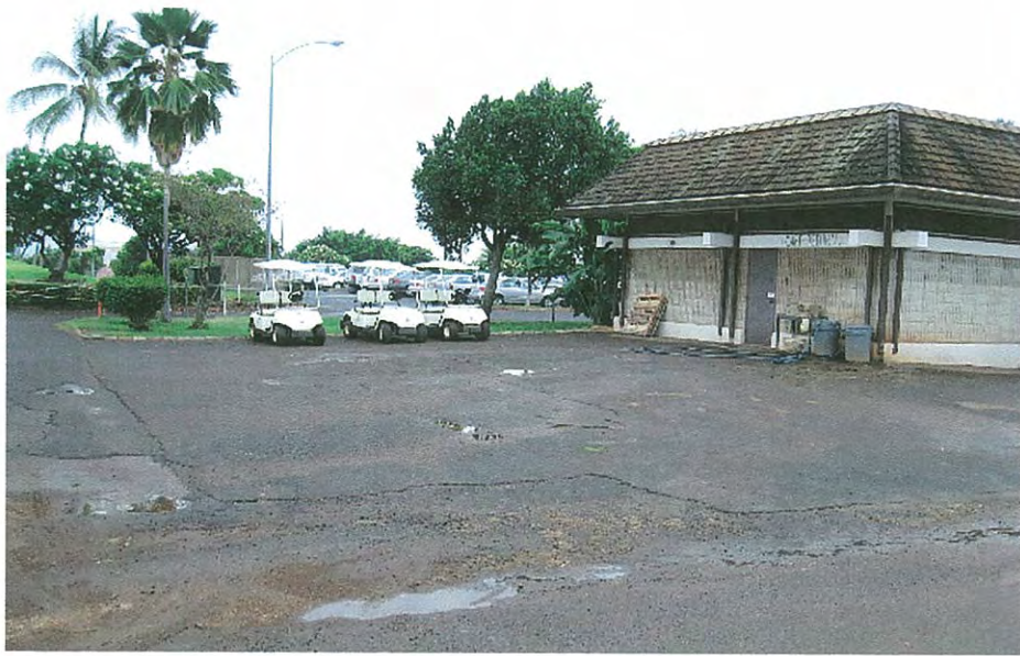
Photograph 1. Cart Wash and Return Area.
