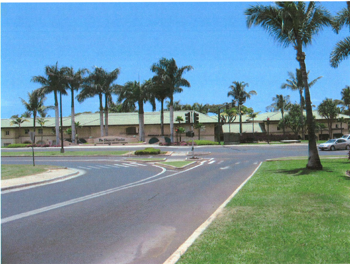
PHOTO NO. 4 - Intersection - View West (Shops at Wailea)
