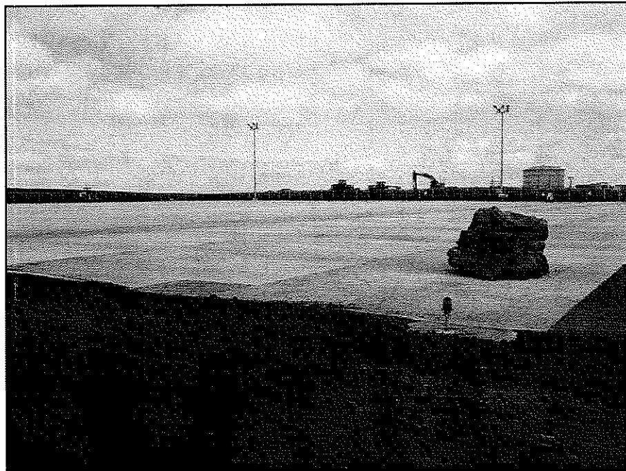
Figure 6. Runway apron extension from east corner, view to west.
