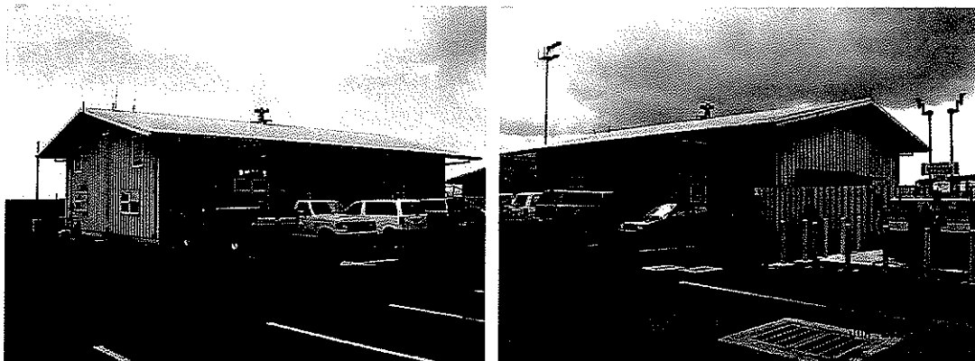
Figures 3 and 4. Existing LNY ARFF Building (Back)
