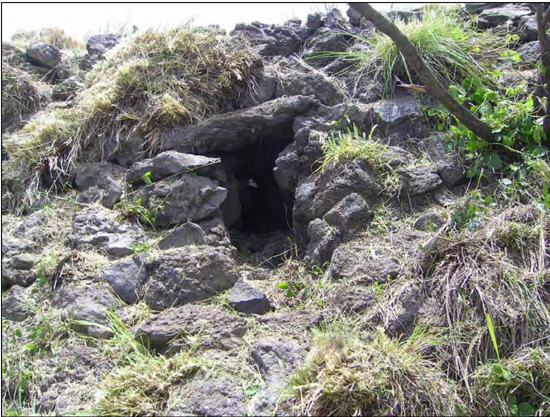
Figure 25: Site 20855, Feature 2 Culvert, View to South.
