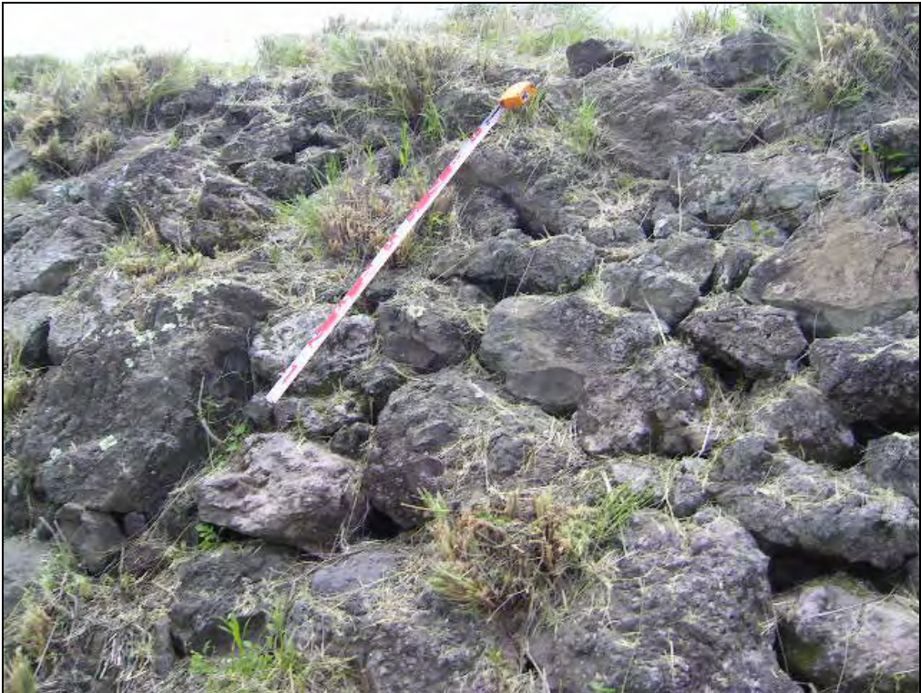
Figure 22: Site 20855 Feature 1 Construction, View to Southeast (1m scale).
