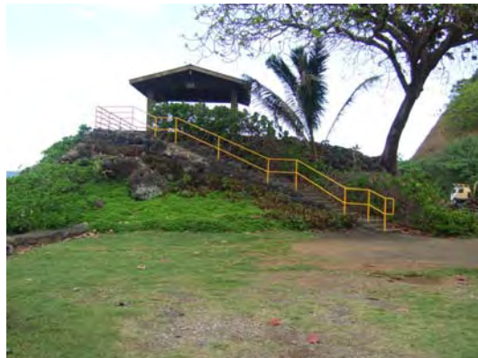
North view of lower pavilion
