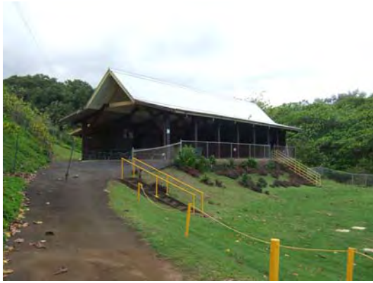
Southwest view of upper pavilion
