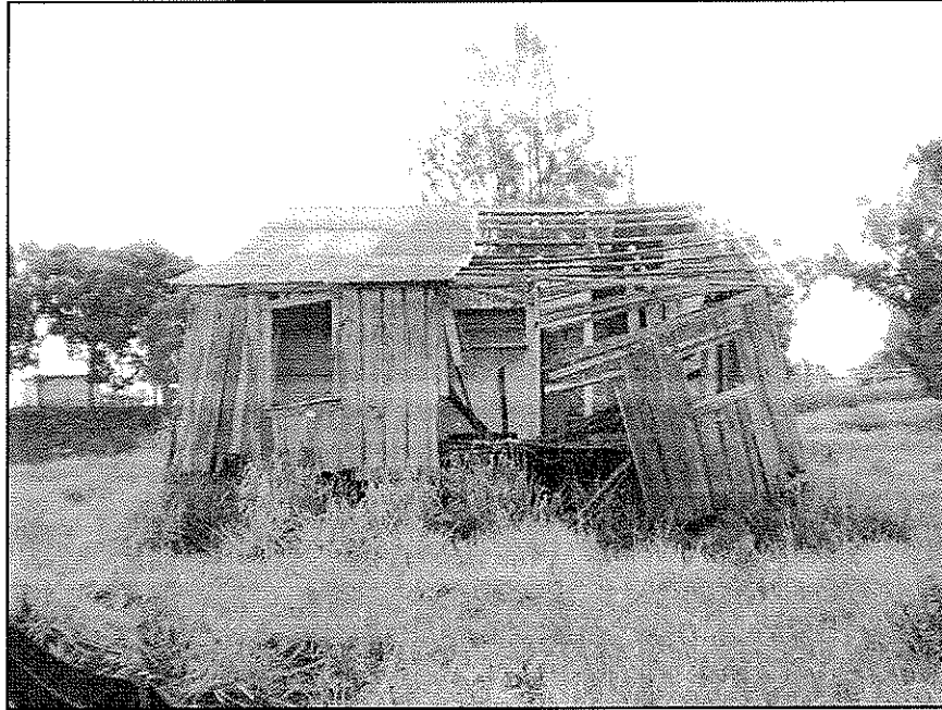
Figure 31. CSH-3, back of structure, view to north.
