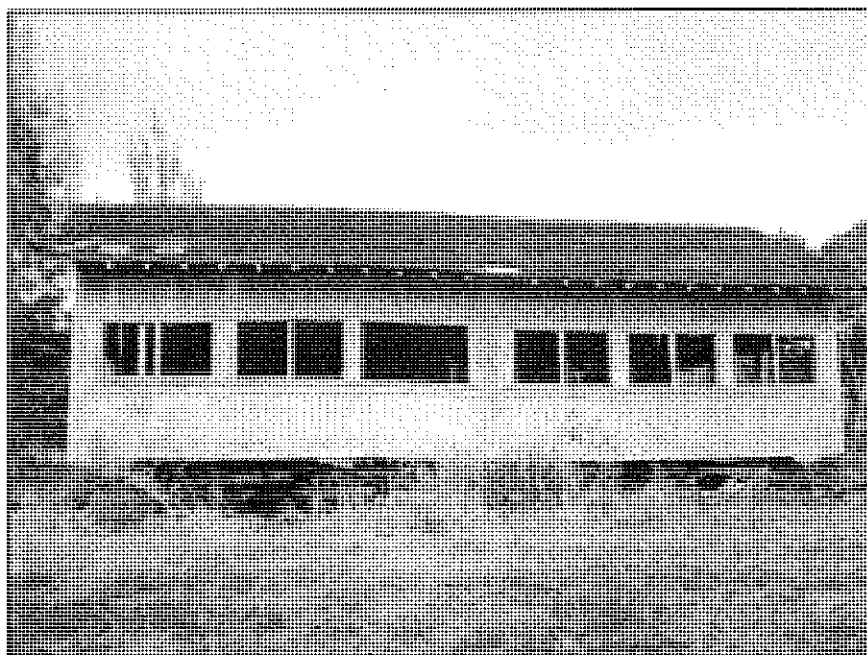
Figure 25. CSH-2, back of structure, view to south.
