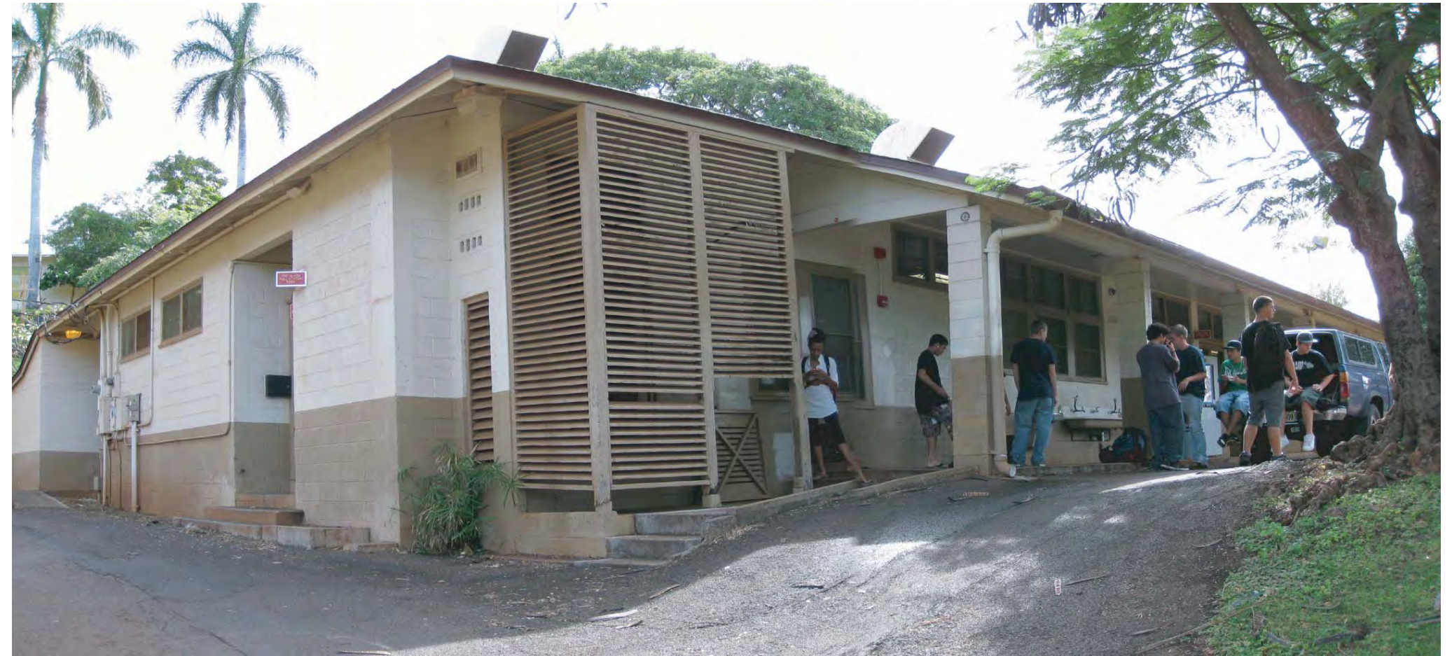
Photo 9. Existing cafeteria, facing mauka from South-Southwest corner of project site.
