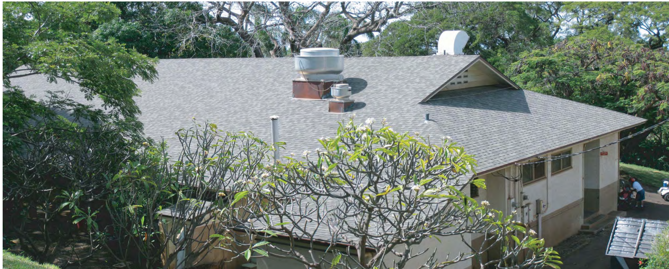
Photo 10. Makai view from shop building above project site; existing cafeteria in foreground.
