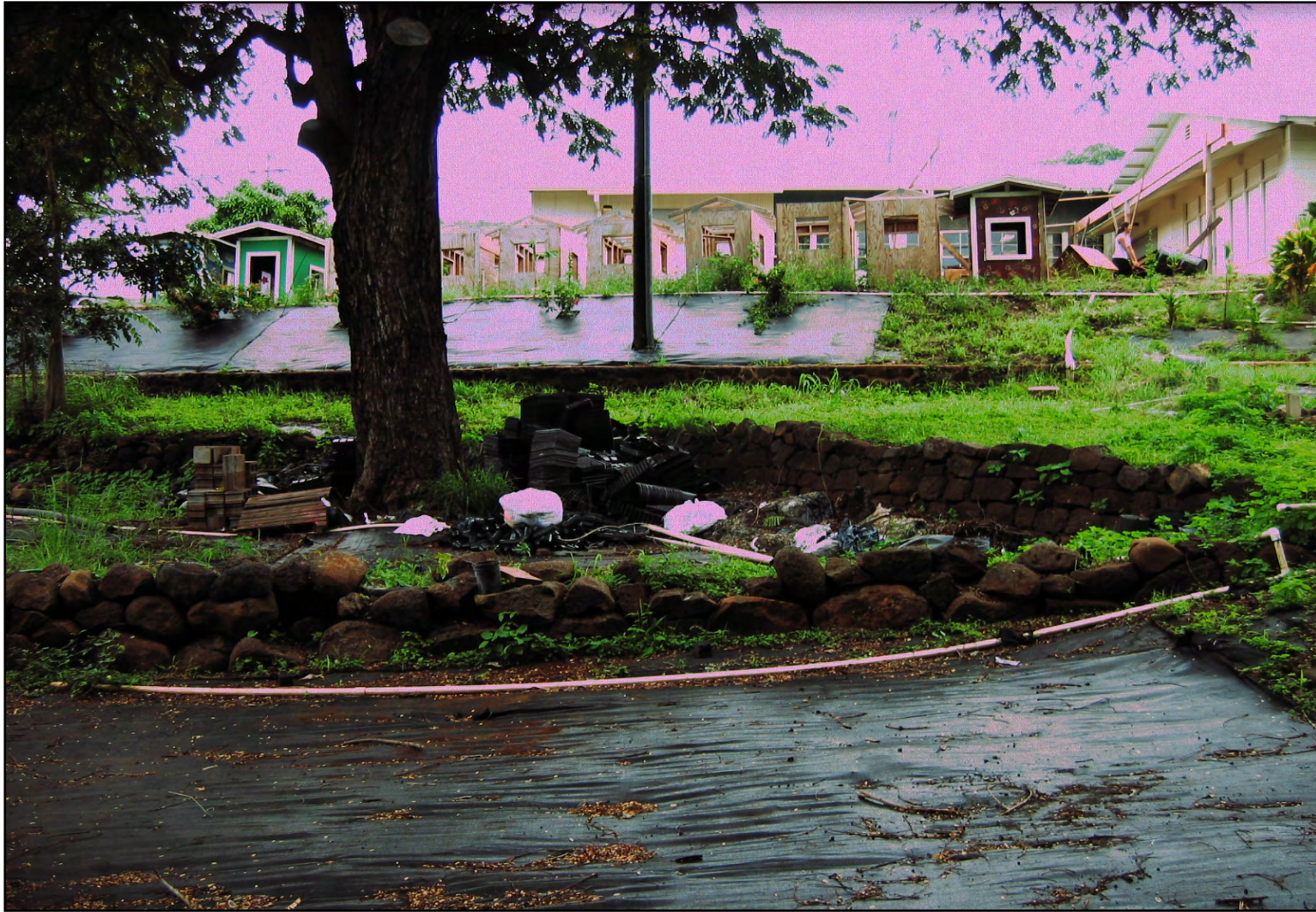
Figure 4: View East of Cut Basalt Terrace Wall
