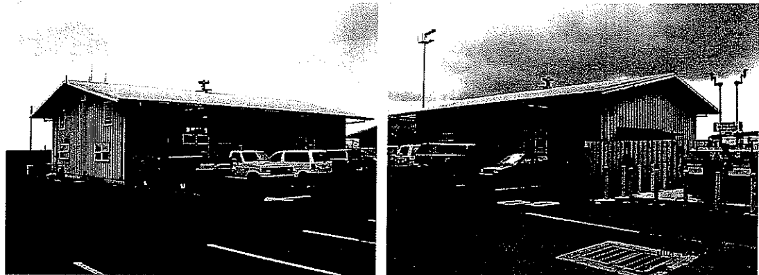
Figures 3 and 4. Existing LNY ARFF Building (Back)
