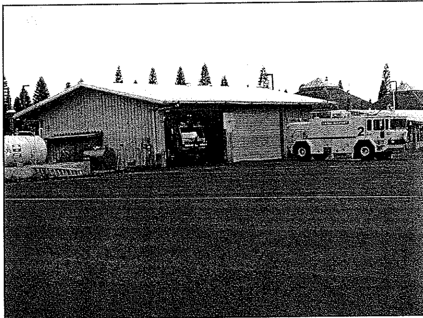
Figure 4. Existing ARFF at the Lāna'i Airport, view to north
