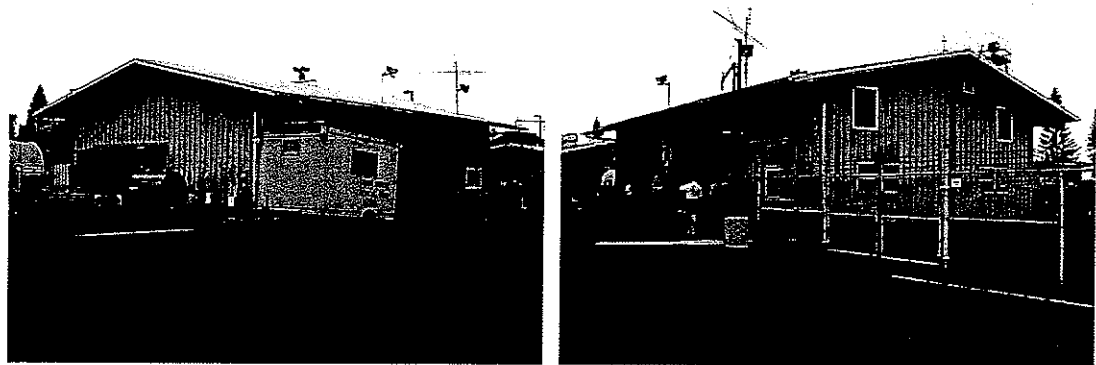
Figures 1 and 2. Existing LNY ARFF Building (Front)
