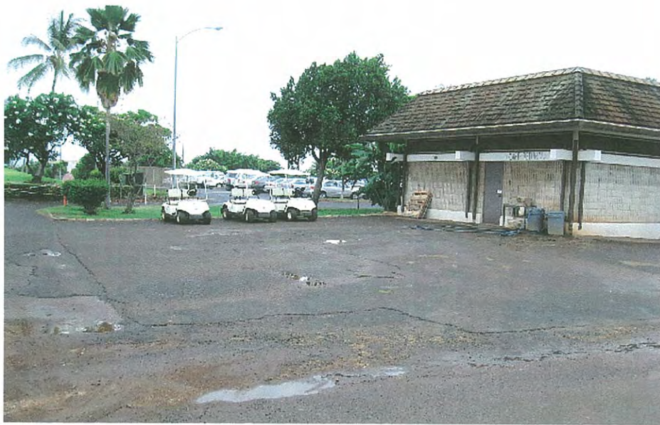
Photograph 1. Cart Wash and Return Area.
