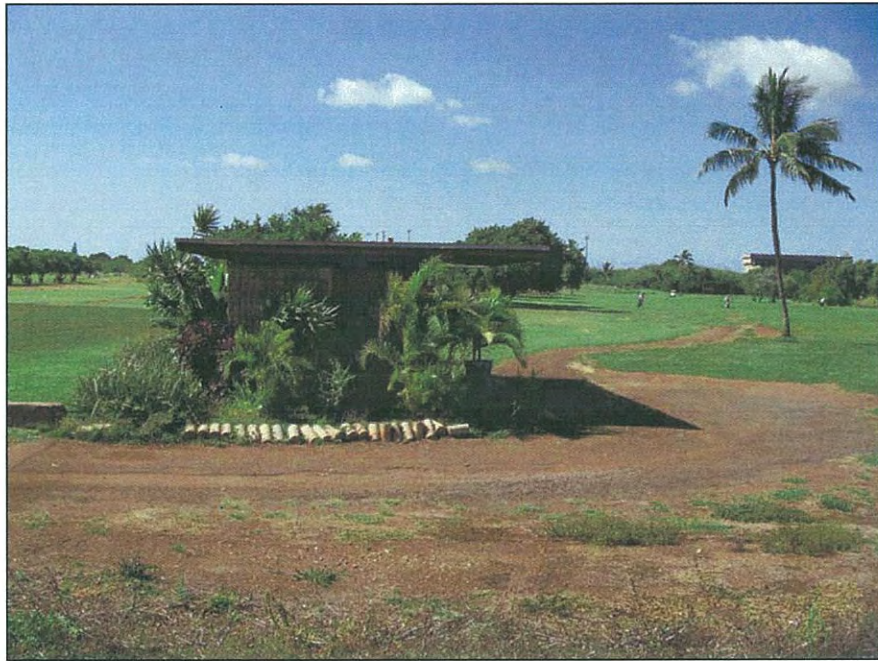
Figure 28. Photograph of restroom facility situated atop LCAs within the northwestern corner of the project area.
