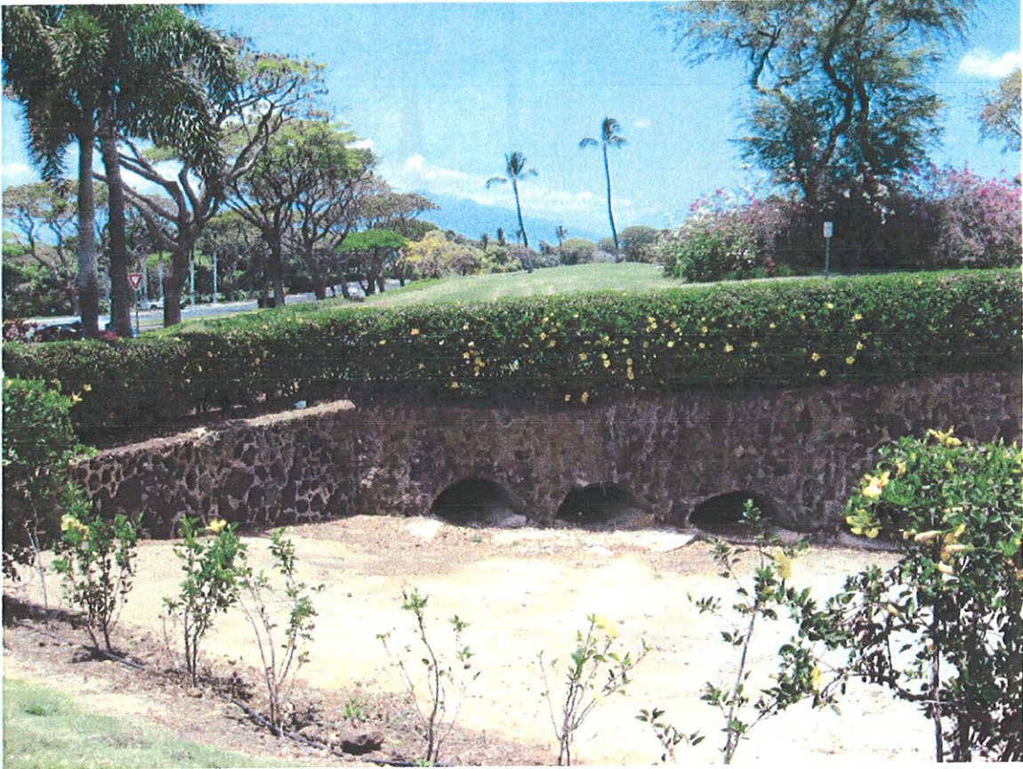
PHOTO NO. 5 - Drainage in Wailea Ike Drive Median
