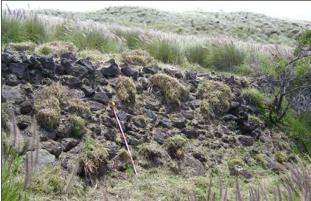
Figure 24: Site 20855, Feature 2, View to Southwest (1m scale).
