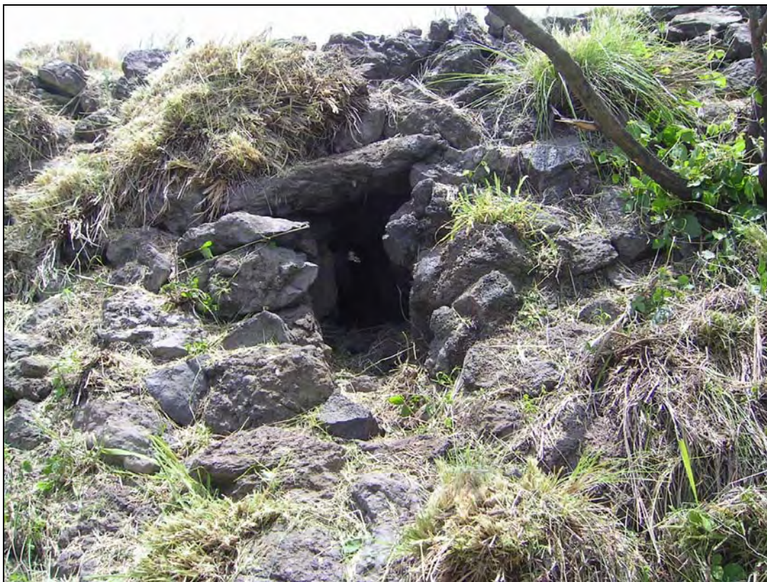
Figure 25: Site 20855, Feature 2 Culvert, View to South.
