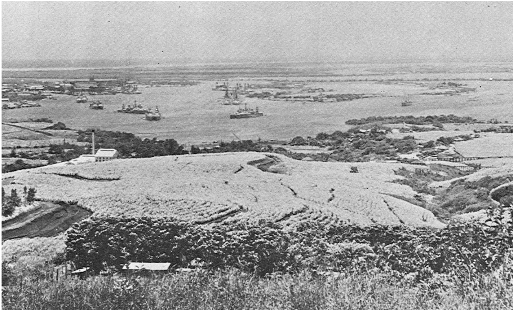
Figure 12. 1932 photograph of Pearl Harbor with the 'Aiea sugar mill in the foreground (Scott 1968:822)
