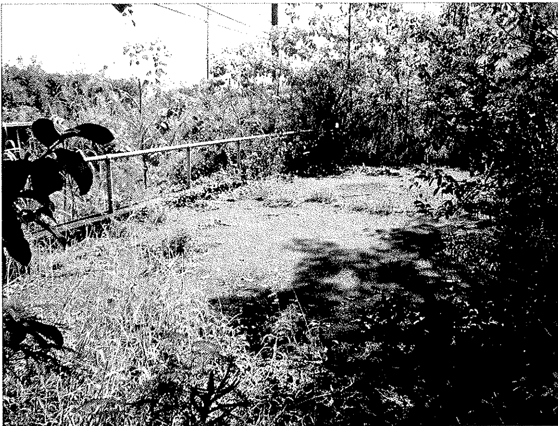
Figure 15. Surface of Bridge showing Guardrails, view to southeast
