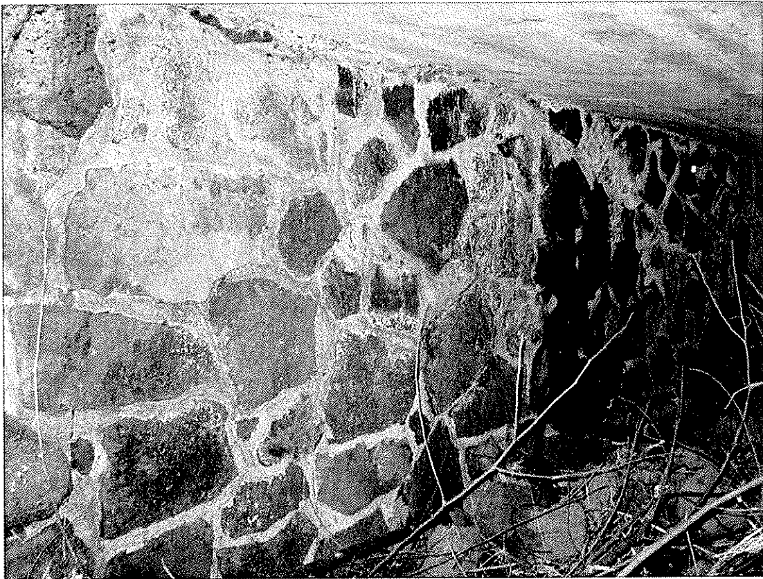
Figure 13. Stone Retaining Wall, view to northwest
