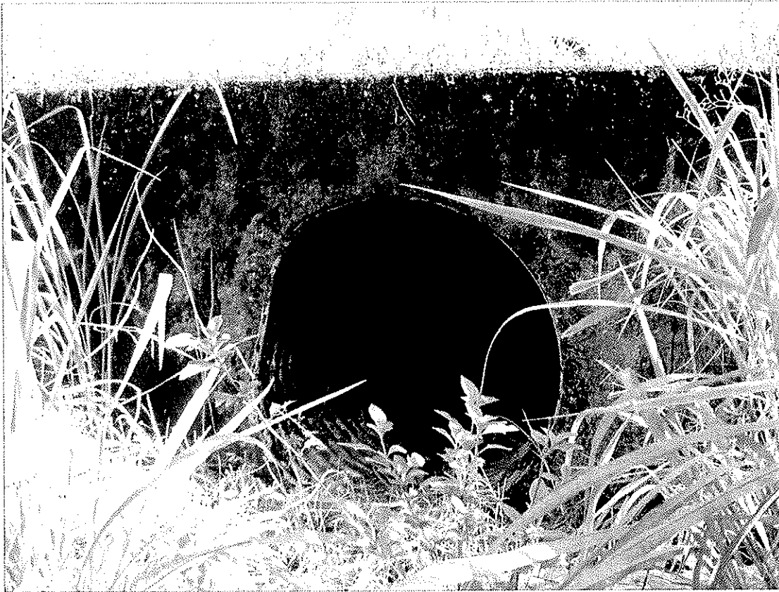
Figure 4. Modern Culvert, view to northeast
