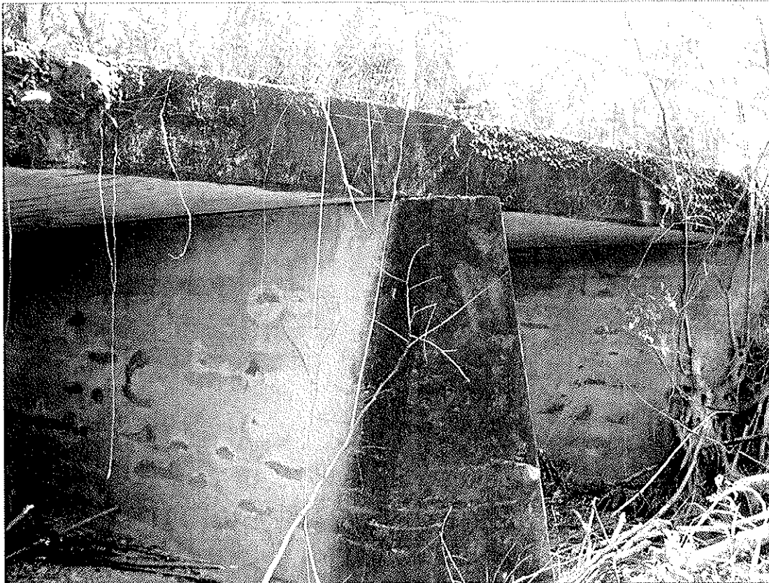
Figure 14. Formed Concrete Piers, view to east
