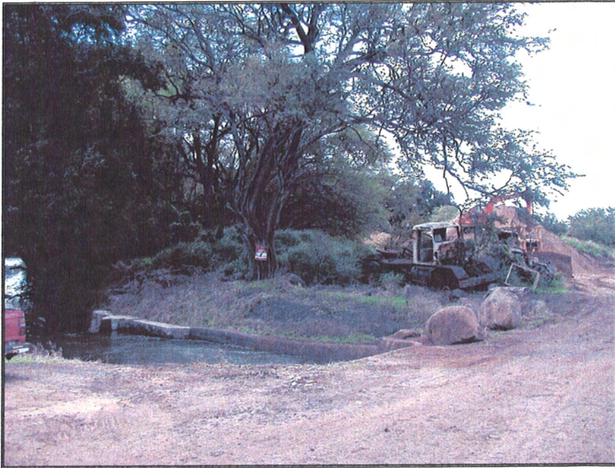
Photograph 1: View to the southeast across intake in left foreground. Project area southeast of equipment.
