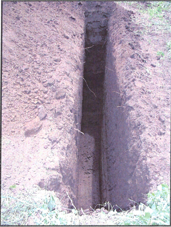
Photograph 5: View to the north of BT 1.
