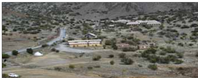
Hale Pōhaku: Keck construction dorms and Subaru construction cabins in foreground, MKSS cafeteria in background.
