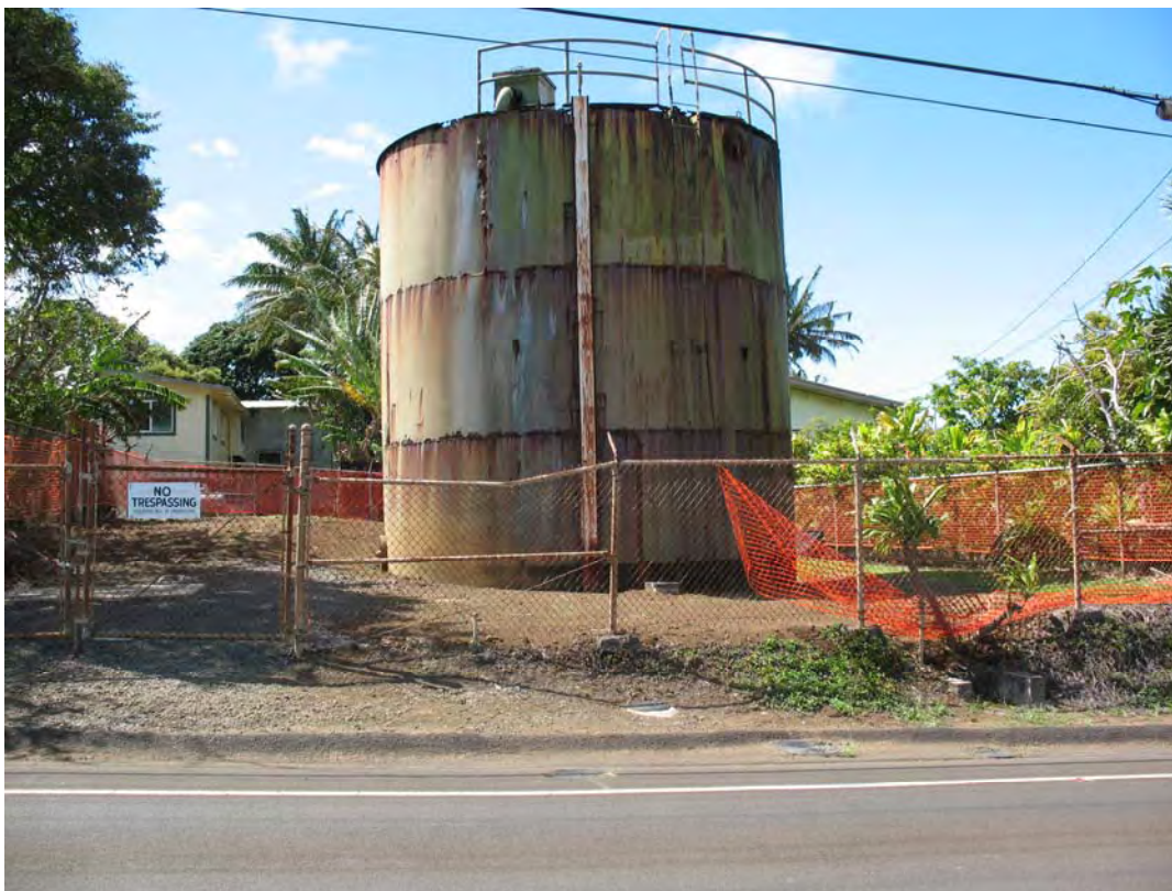
Figure 5. Existing tank on Parcel 3-5-4-11:099, view to the west.
