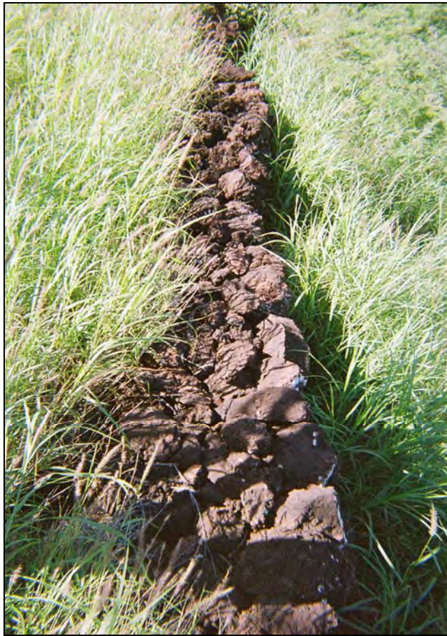
Figure 21: Photograph of Site -6241, Top of Wall Overview. View to West.
