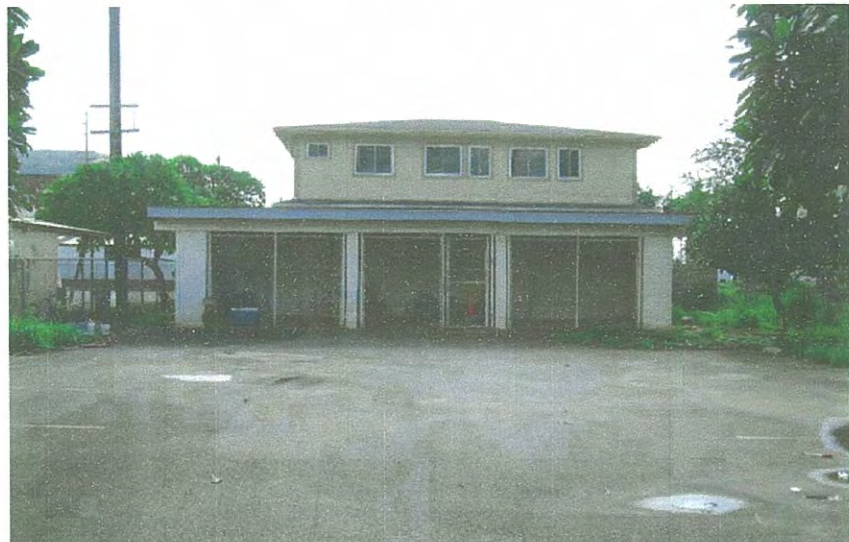
Photograph 3. Secured Storage Shed. Note 2-story Dwelling Behind the Shed.
