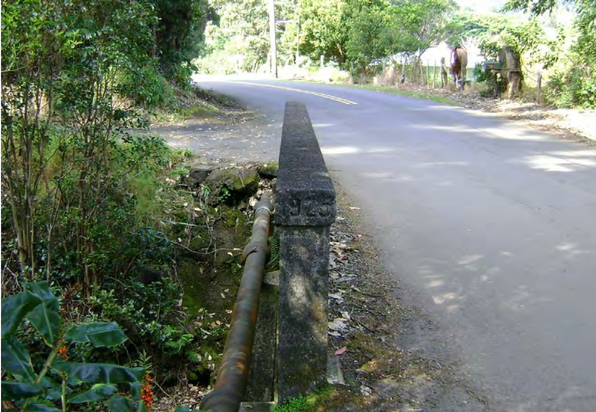
Photo 2a. The pipeline will cross streams attached to bridges, as currently ▲
