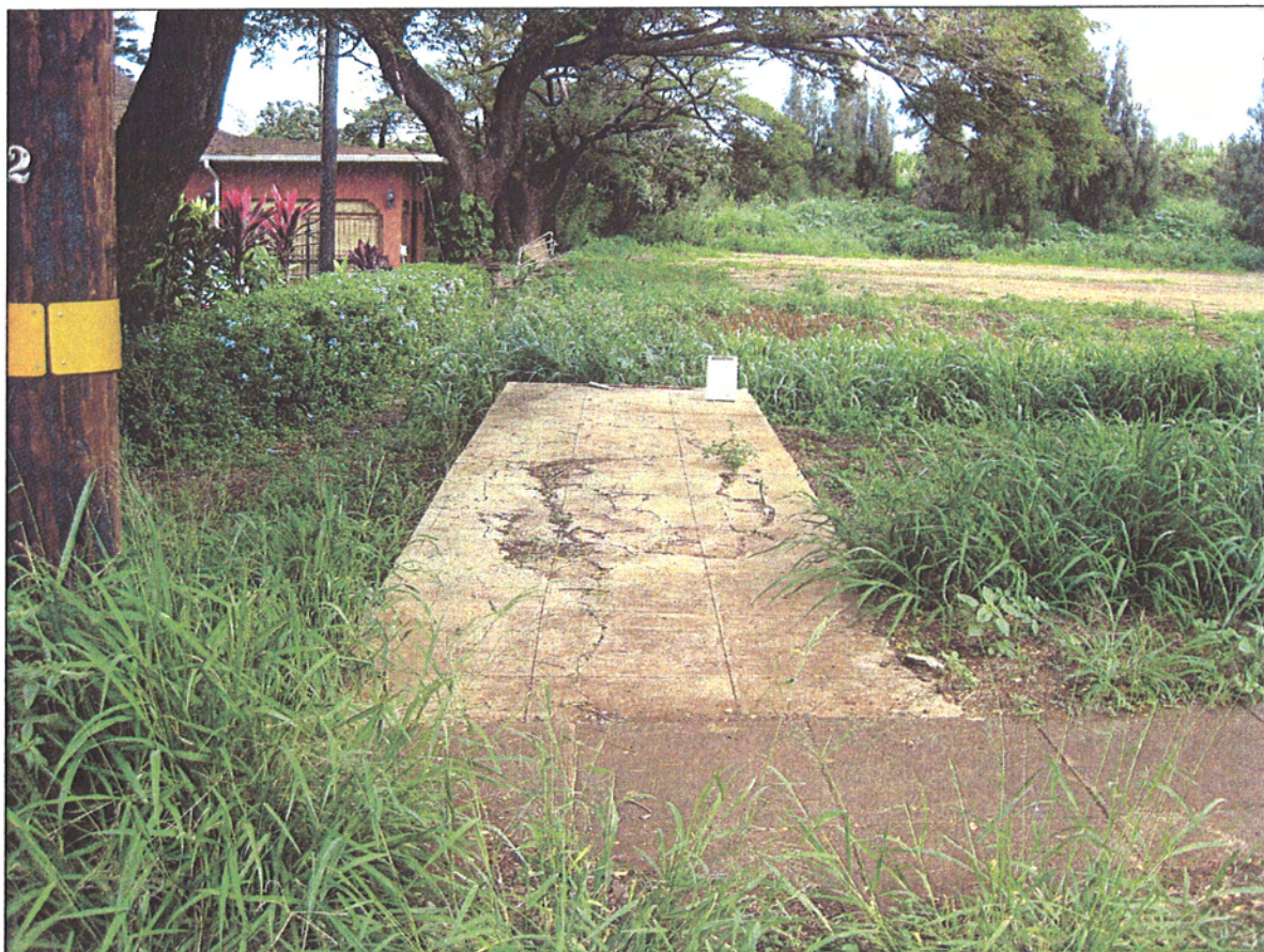
Figure 8: Site -6427, Feature A. Concrete Ramp. View to Northeast.
