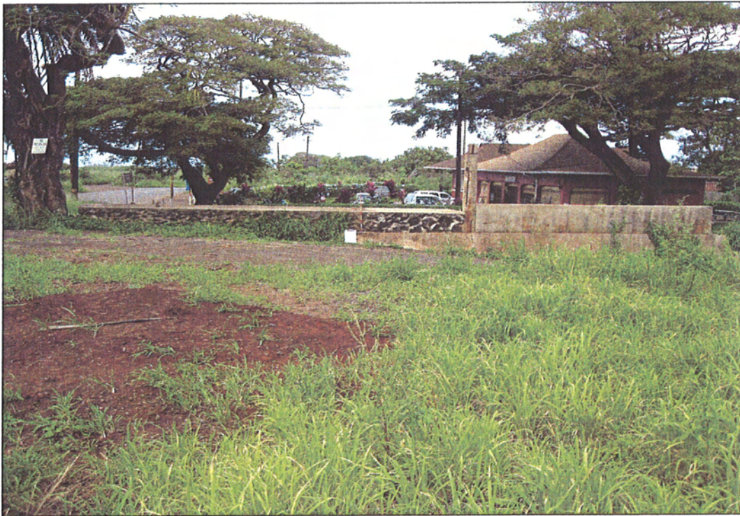
Figure 10: Site -6427, Feature C. Rock/Concrete Wall. View to Southeast.
