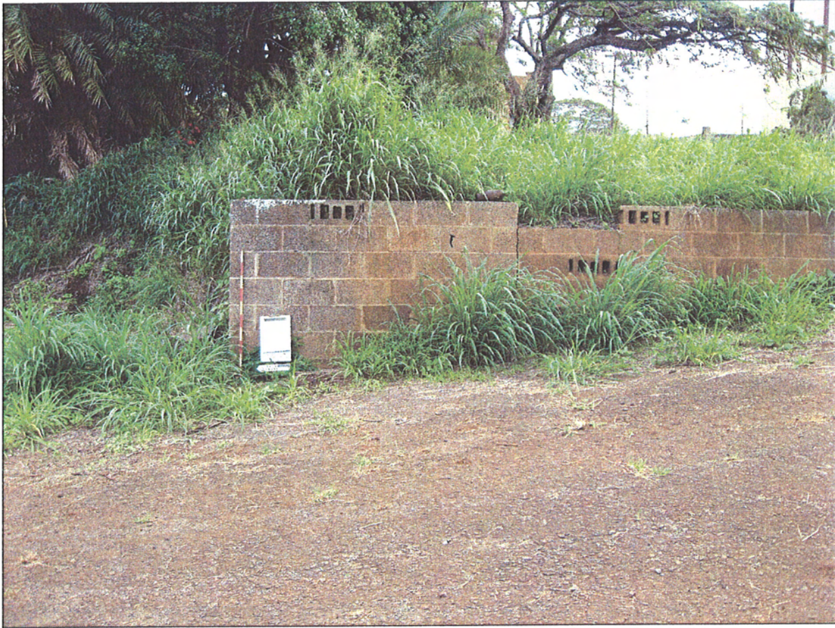
Figure 13: Site -6427, Feature E. Tile and Mortar Wall. View to Southeast.
