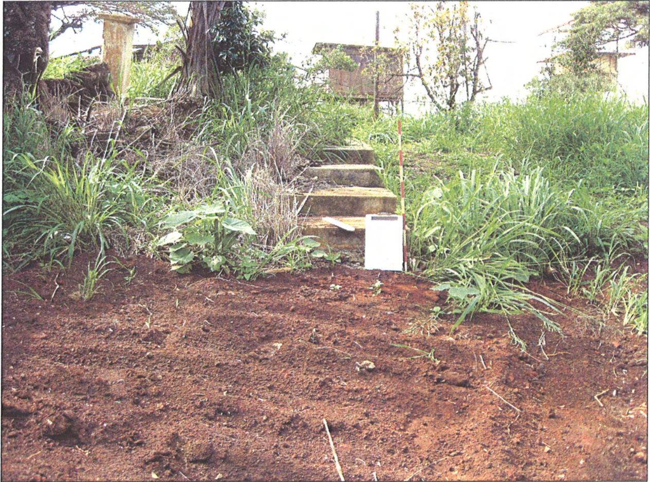
Figure 9: Site -6427, Feature B. Concrete Stairs. View to Southwest.
