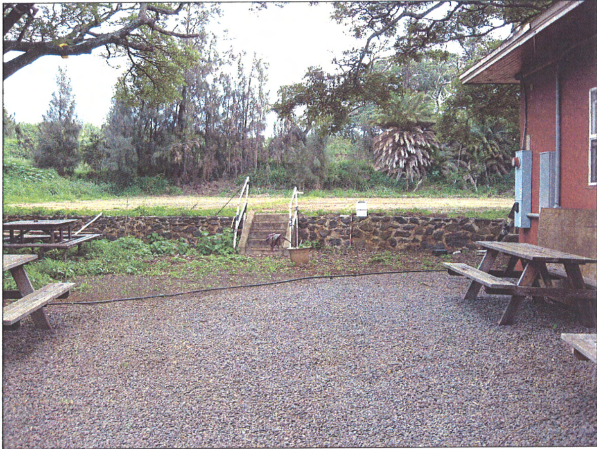
Figure 16: Site -6427, Feature I. Rock Retaining Wall with Stairs. View to Southeast.
