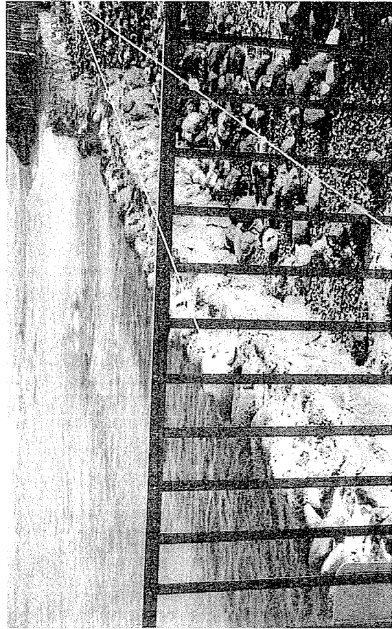
Photos depict the seawall fronting the Hale Kai complex. It appears that an additional layer of rocks has been cemented onto the top of the wall in an attempt to elevate the wall's current height.
