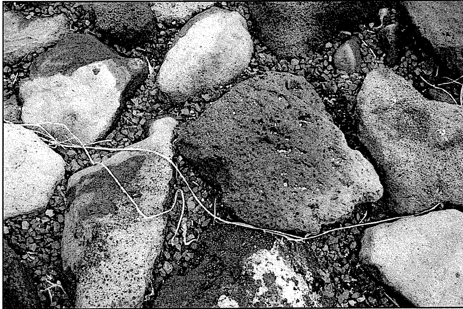
Figure 8. Crest stones on repair section
