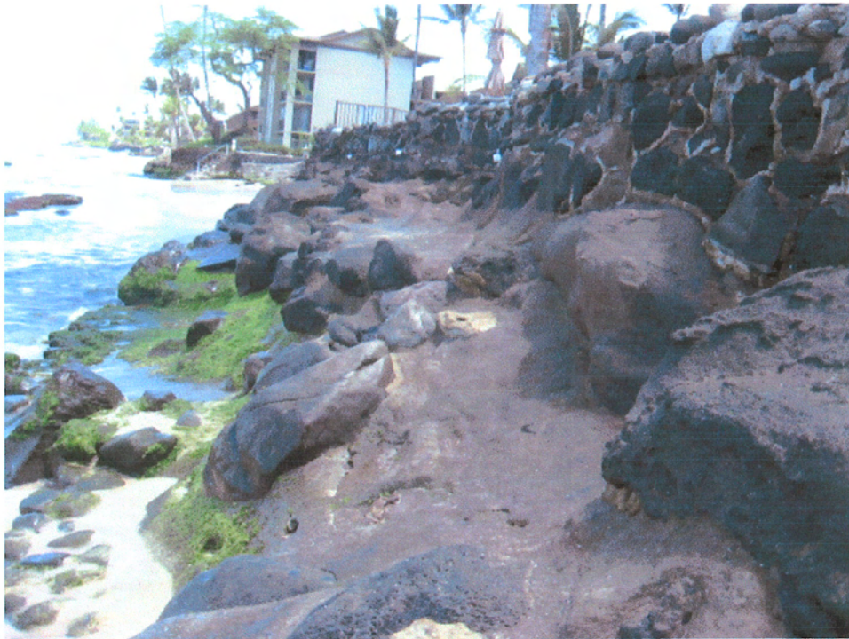
Existing Seawall Structure
