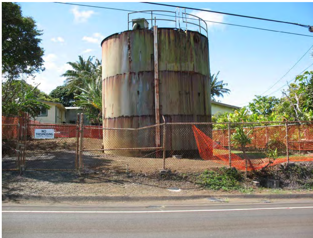
Figure 5. Existing tank on Parcel 3-5-4-11:099, view to the west.
