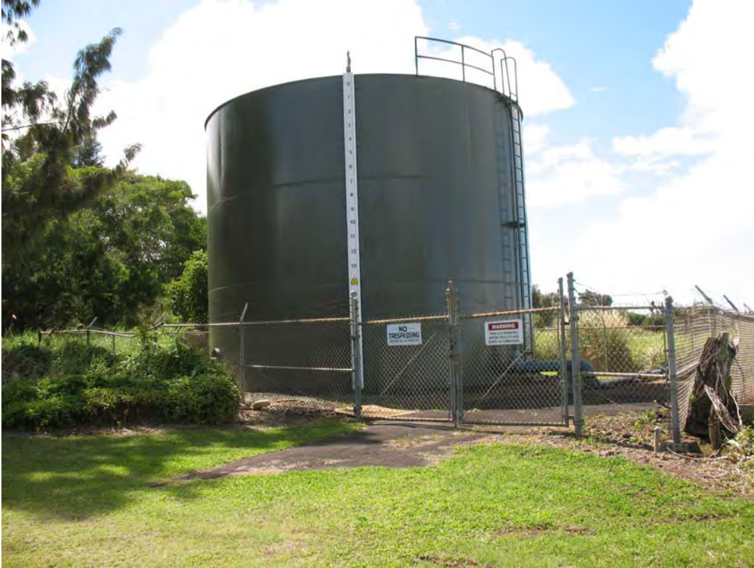
Figure 6. Existing tank on Parcel 3-5-4-02:008, view to the west.
