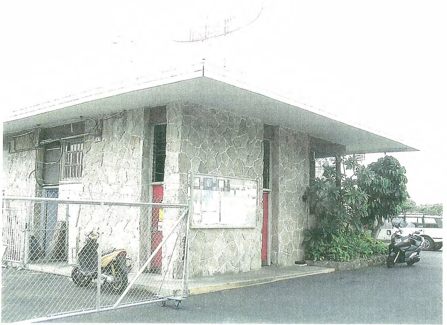
Photo 2C - Fuel Dock Site. View of existing structure on property.
