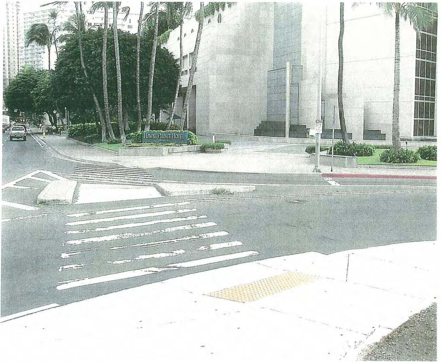
1F - View from Ewa corner of Ala Moana Blvd. and Holomoana St. looking Diamond Head. Hawaii Prince Hotel is in the background.
