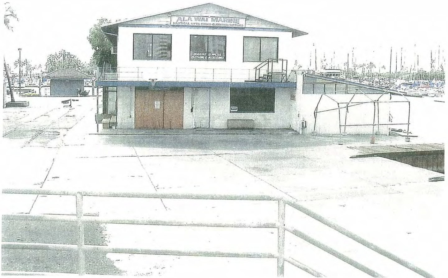
Photo 11 - Boatyard Repair Site. View of existing structure from Ewa-Mauka corner of property looking Makai.
