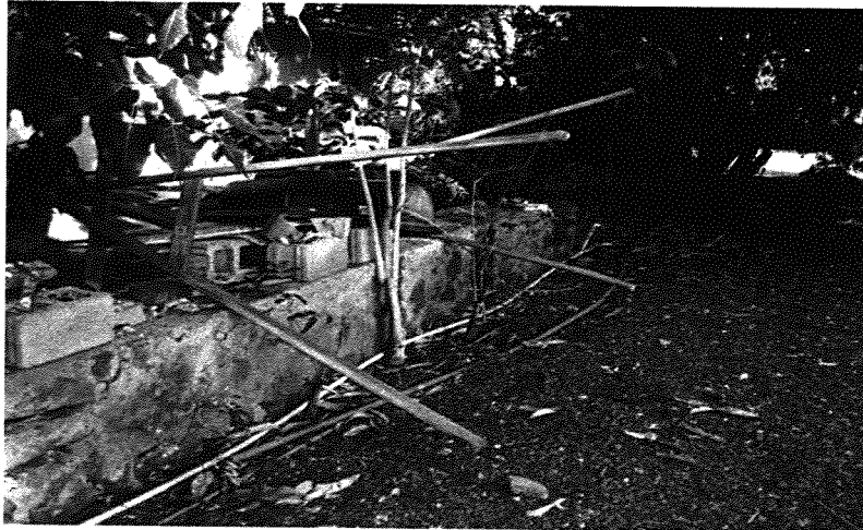
Photograph 6: Overview of Site 6661 wall section, view to SE.
