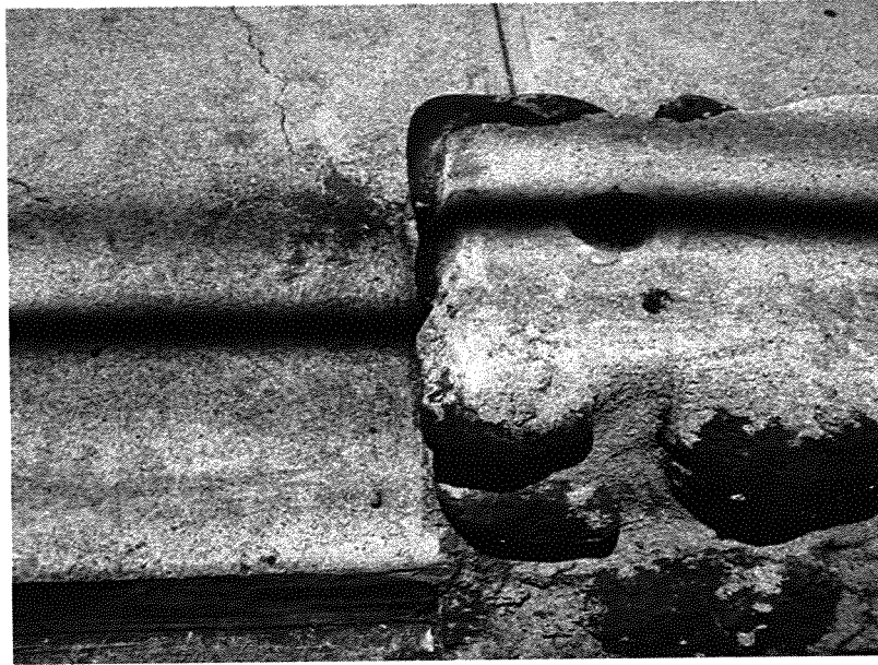
Photograph 3: Site 6660 rock wall showing rail insertion hole.
