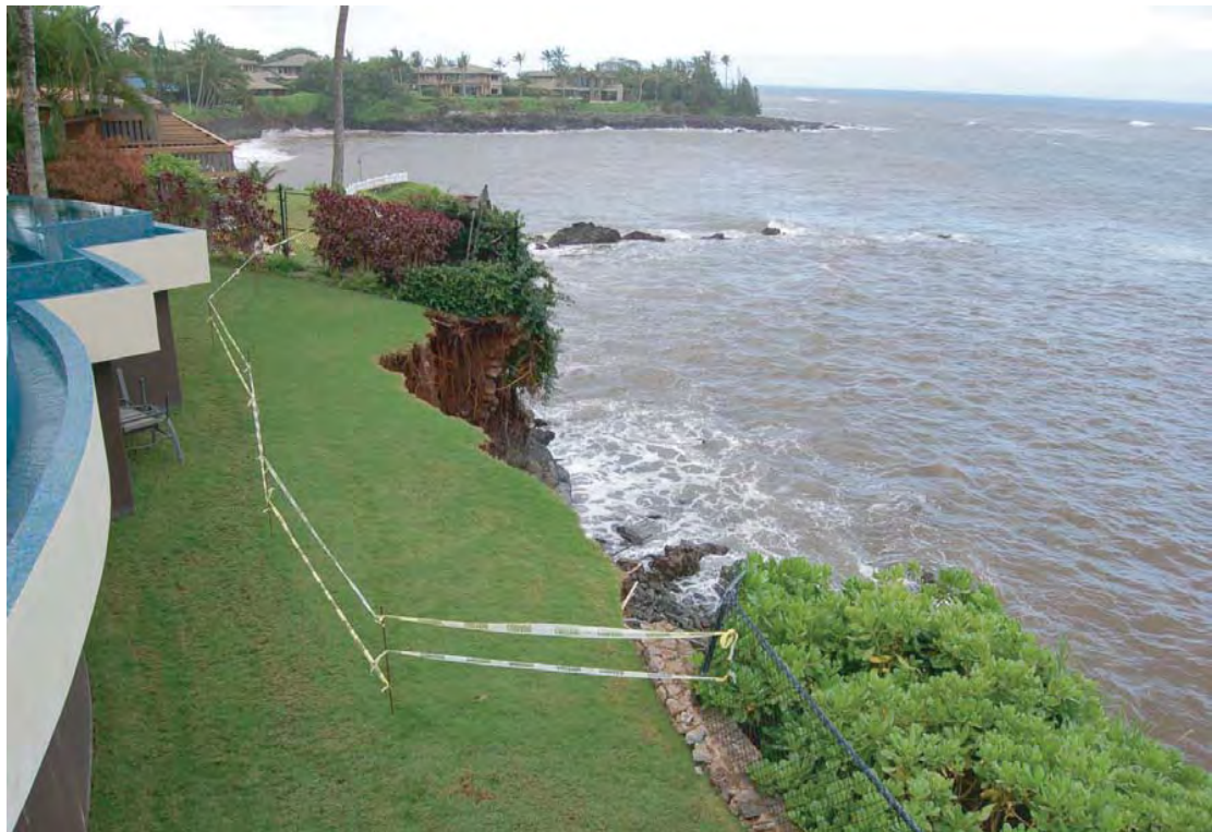
3. View from above, showing top of failed slope and edge of pool
