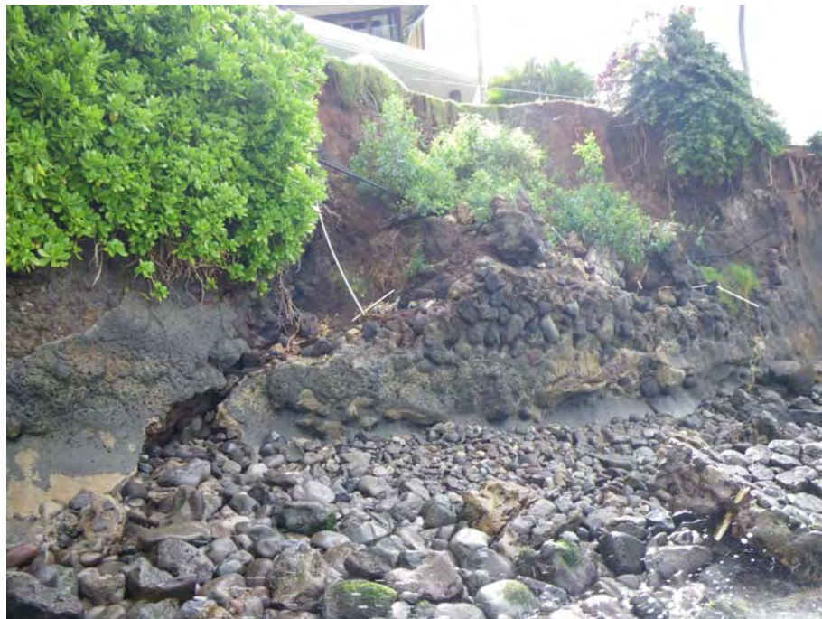
Figure 5: View East of Collapsed Seawall
