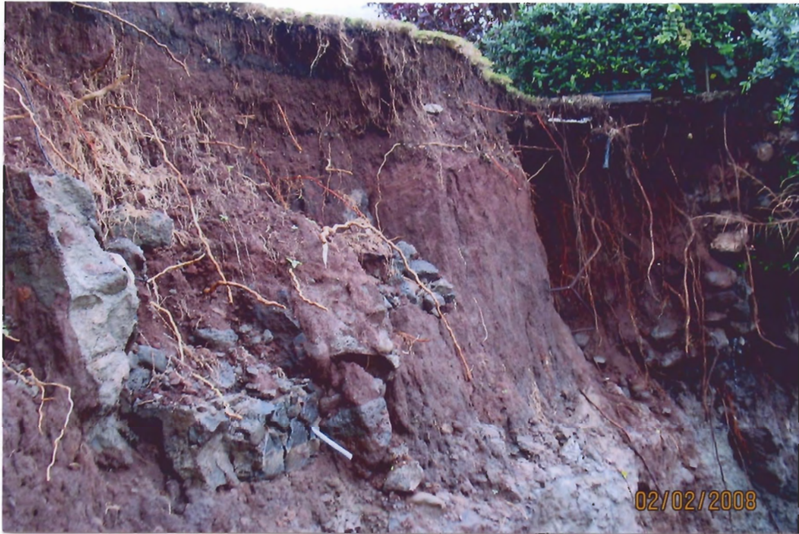
Close Up View of Slope Failure
