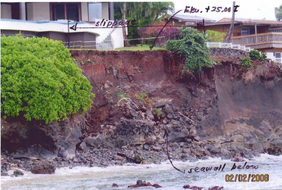
2 Elevation View of Soil Slippage Area
