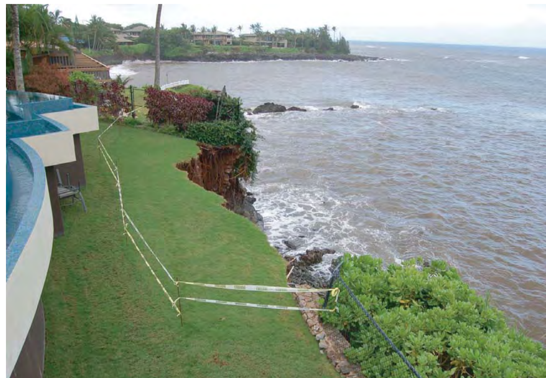
3. View from above, showing top of failed slope and edge of pool
