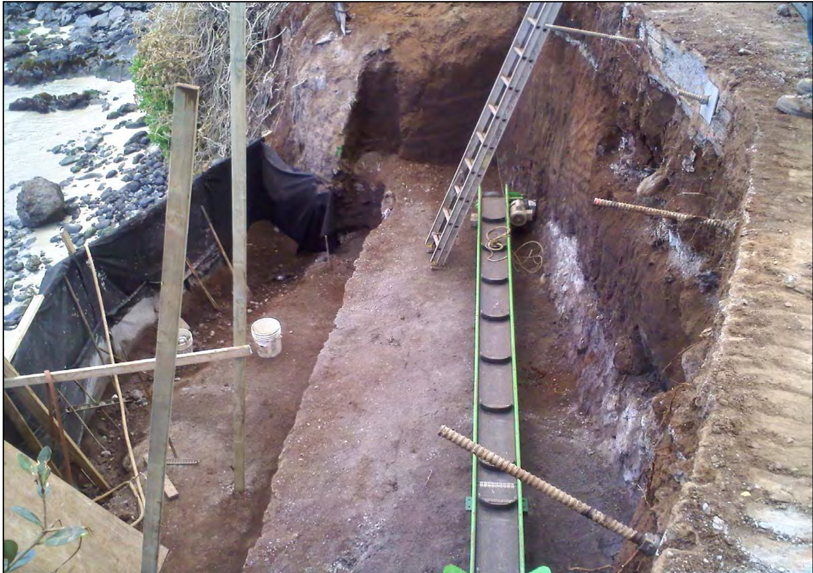
Figure 7: View North of Excavation for New Seawall
