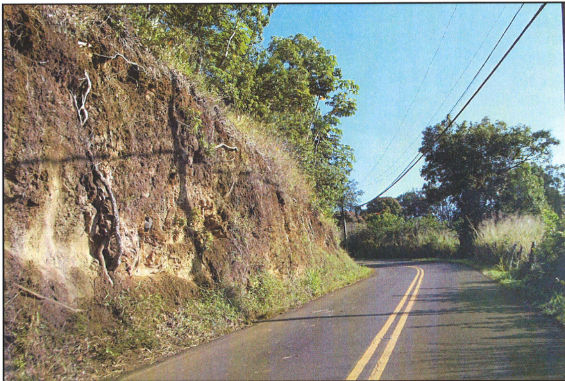
Figure 8: View West of Ha`ikū Road Waterline Corridor Exiting Kuiaha Gulch
