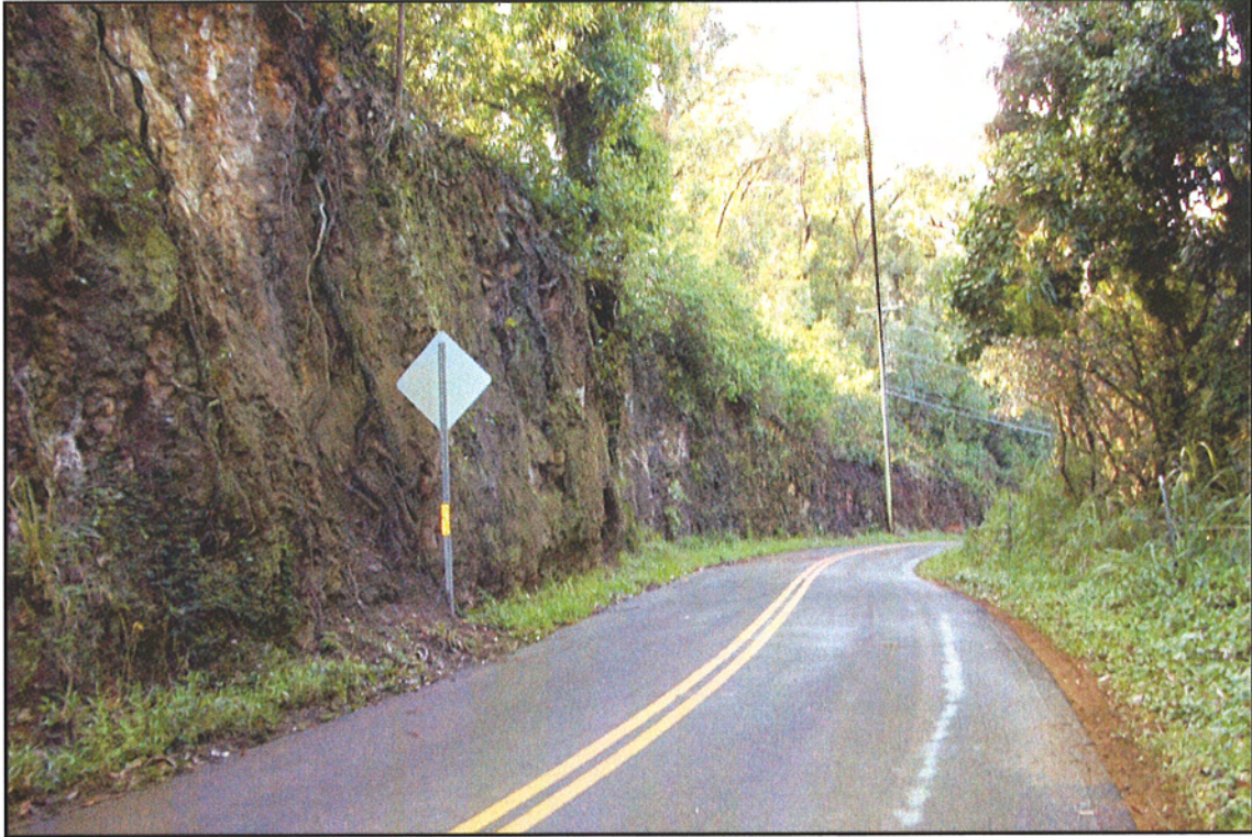
Figure 7: View West of Ha`ikū Road Waterline Corridor Entering Kuiaha Gulch
