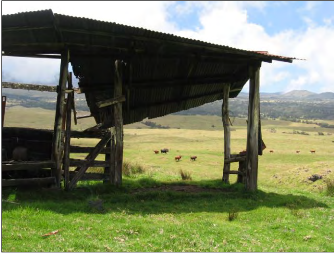
Figure 10. Feature T2 corral, northern portion of structure, view to the west/northwest.
