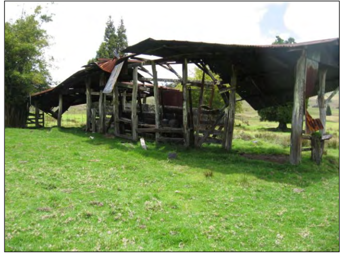
Figure 11. Feature T2 corral, southern portion of structure, view to the south/southwest.
