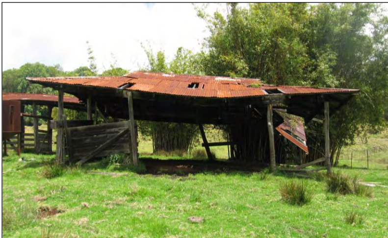
Figure 12. Feature T2 corral, southern portion of structure, view to the east.
