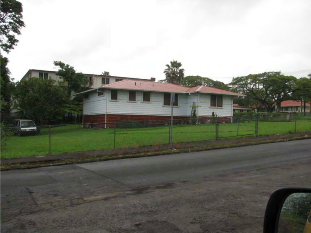
Figure 3 – Project Site Photographs
