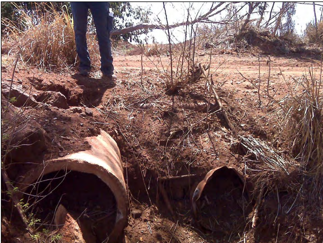
Figure 35. Sub-feature 18, concrete pipe for drainage underneath Old Government Road; view northeast
