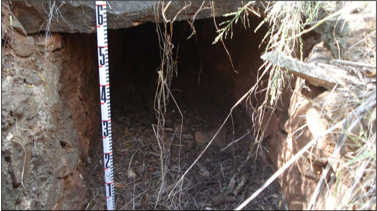
Figure 29. Sub-feature 11, stacked and mortared boulder ditch culvert; view southwest
