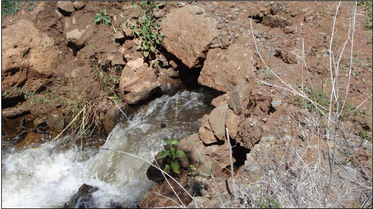
Figure 33. Sub-feature 16, stacked boulder ditch culvert; view north
