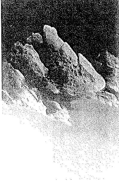
Figure 5. Coral and coralline red algae on seaward face of pile 14A.
