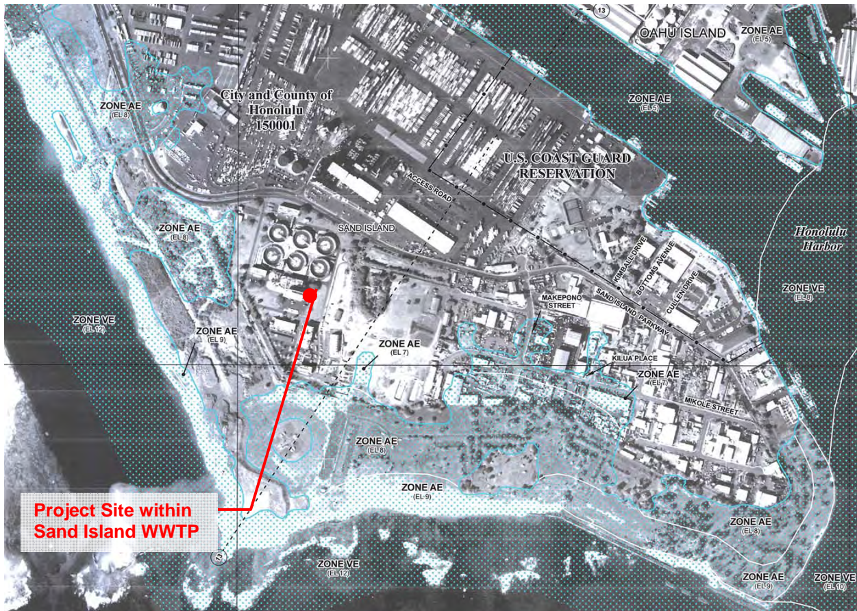
Figure 3-2, Sand Island WWTP, FEMA FIRM Panel 15003C0361G (July 22, 2009)
