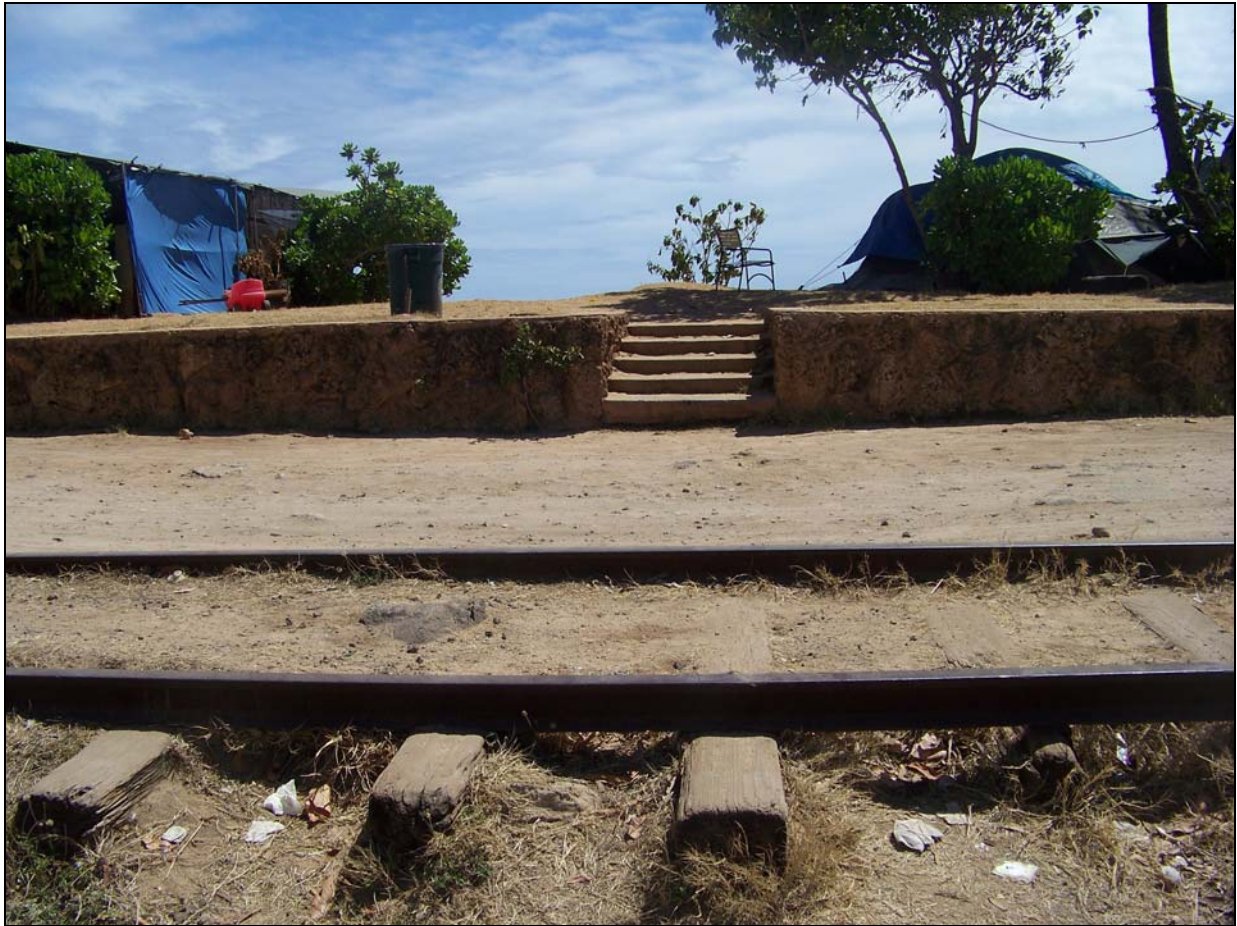
Figure 24. Portion of the OR&L railroad showing rail and ties still in place, view west
