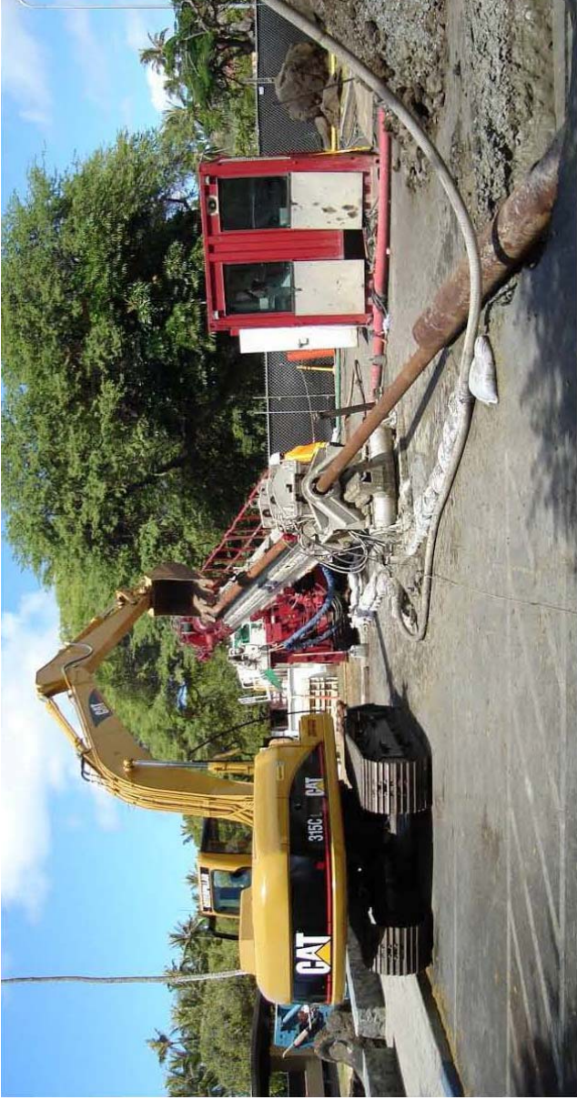
HDD Drill Rig. Control cabin on right. Niu Valley, Hawaii, 2006
