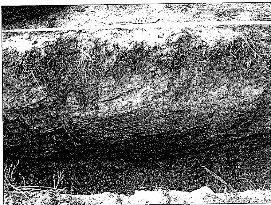
Photo # 11: Overview of the west face wall of BT-10, view to the west.
