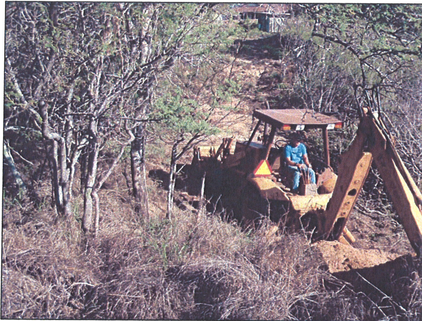
Photo # 28: BT-7 Excavation Overview, View to North.
