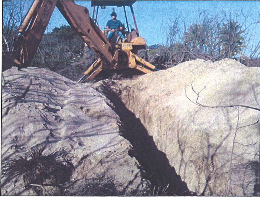
Photo # 26: Overview of BT-6, View to South.
