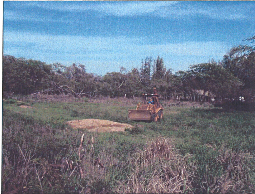
Photo # 42: Backfilling BT-15, View to East.
