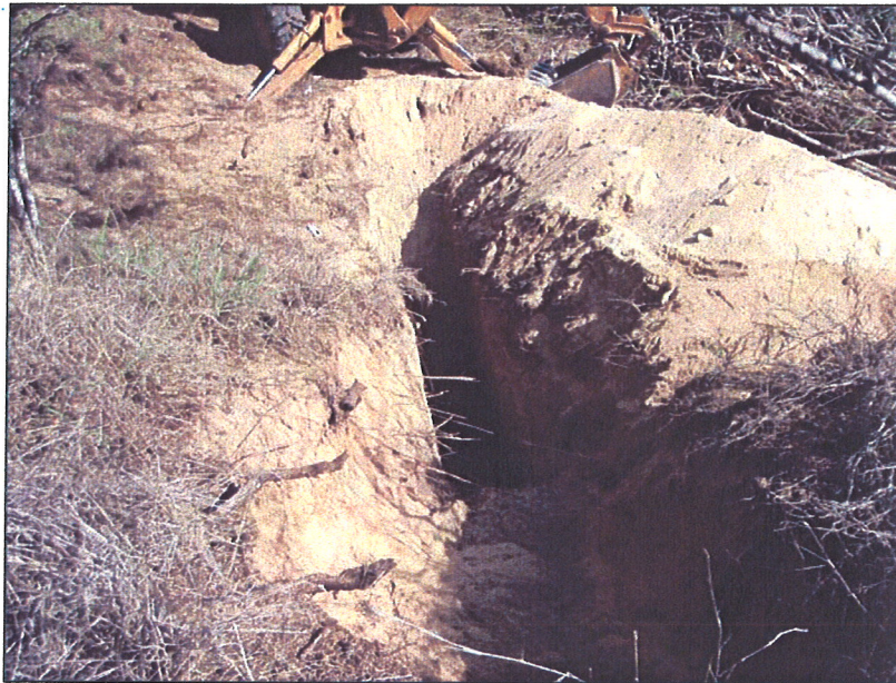
Photo # 31: BT-9 Overview from Top of Slope, View to North.
