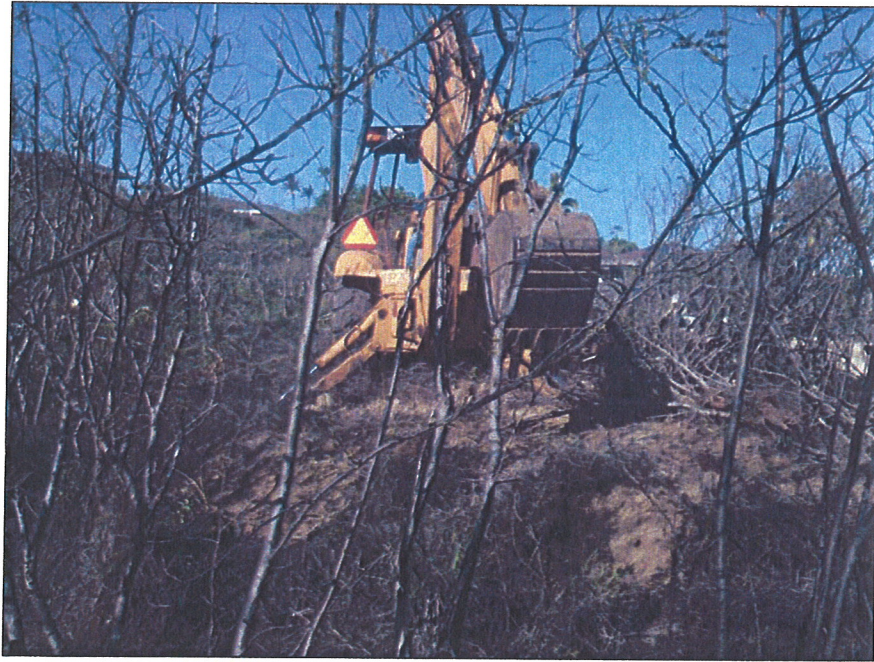
Photo # 45: Pre Excavation Overview of BT-17, View to North.
