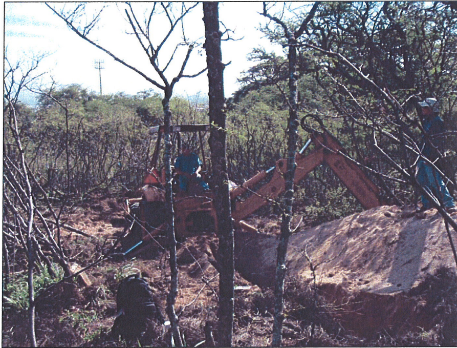
Photo # 36: BT-12 Excavation Overview to East.
