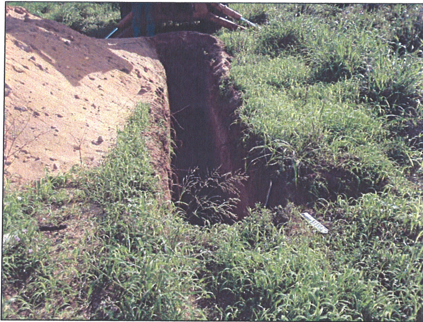
Photo # 40: BT-15 Excavated Trench Overview to South.
