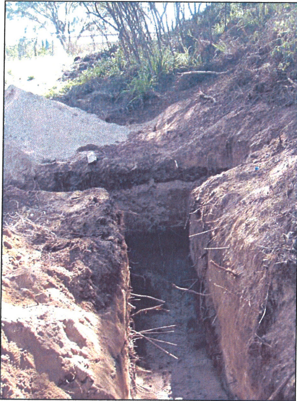
Photo # 24: BT-5 Post-Excavation Overview with BT-5 (foreground) and BT-4 in (background), View to Southeast.
