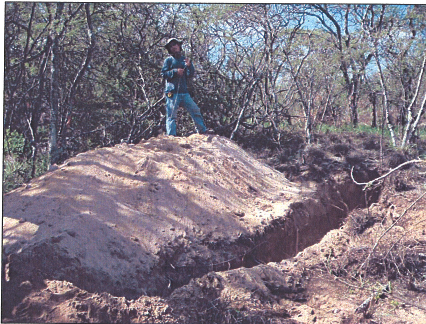
Photo # 34: BT-11 Overview of Excavated Trench, View to Southwest.
