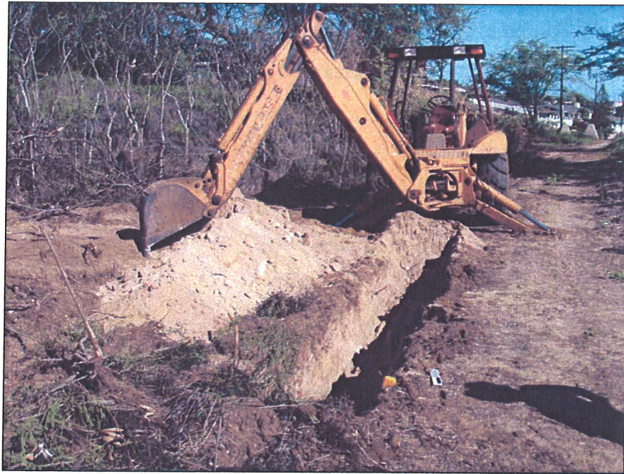
Photo # 20: Post-Excavation of BT-3, View to North.
