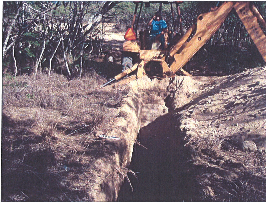
Photo # 38: Overview of BT 13, View to East.
