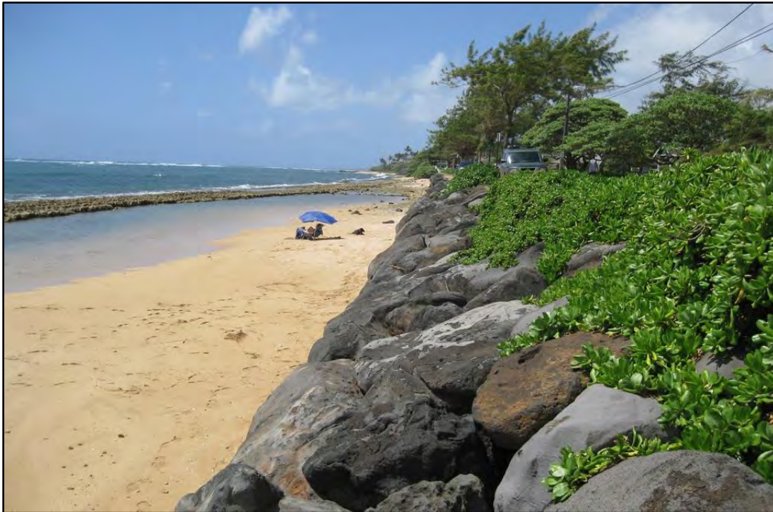
Figure 2-4 View of beach, revetment and protected swimming area in northern reach
