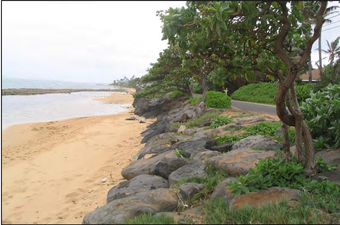
Figure 2-24 A 2004 photo showing the intact revetment between Stations 9+70 to 10+30
