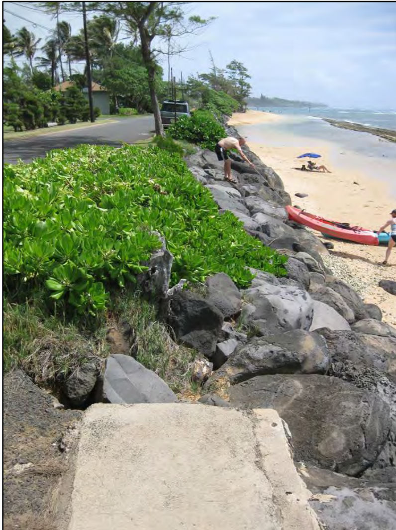
Figure 2-15 End of concrete cap, start of revetment, Station 5+70
