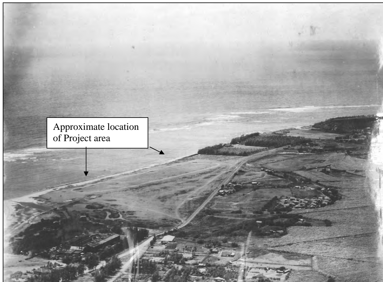
Figure 11. 1924 aerial photograph of Kapa'a showing the Project area vicinity. The area is described as cleared "for future subdivision" (Fernandez 2009:113). Hawaiian Canneries Company Limited. is in foreground, makai of highway
