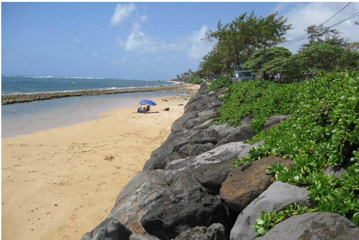
Photo 5: View of beach, revetment and protected swimming area in northern reach (Source: Sea Engineering, Inc., 2011)
