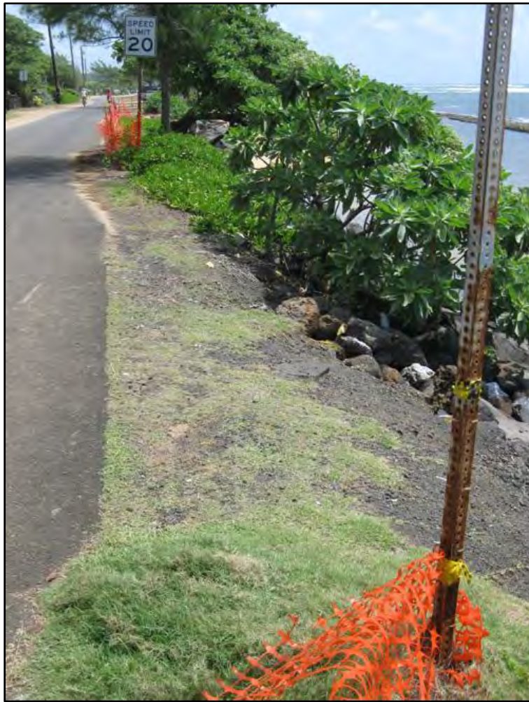
Figure 2-20 Narrow road shoulder between Stations 8+40 and 8+80
