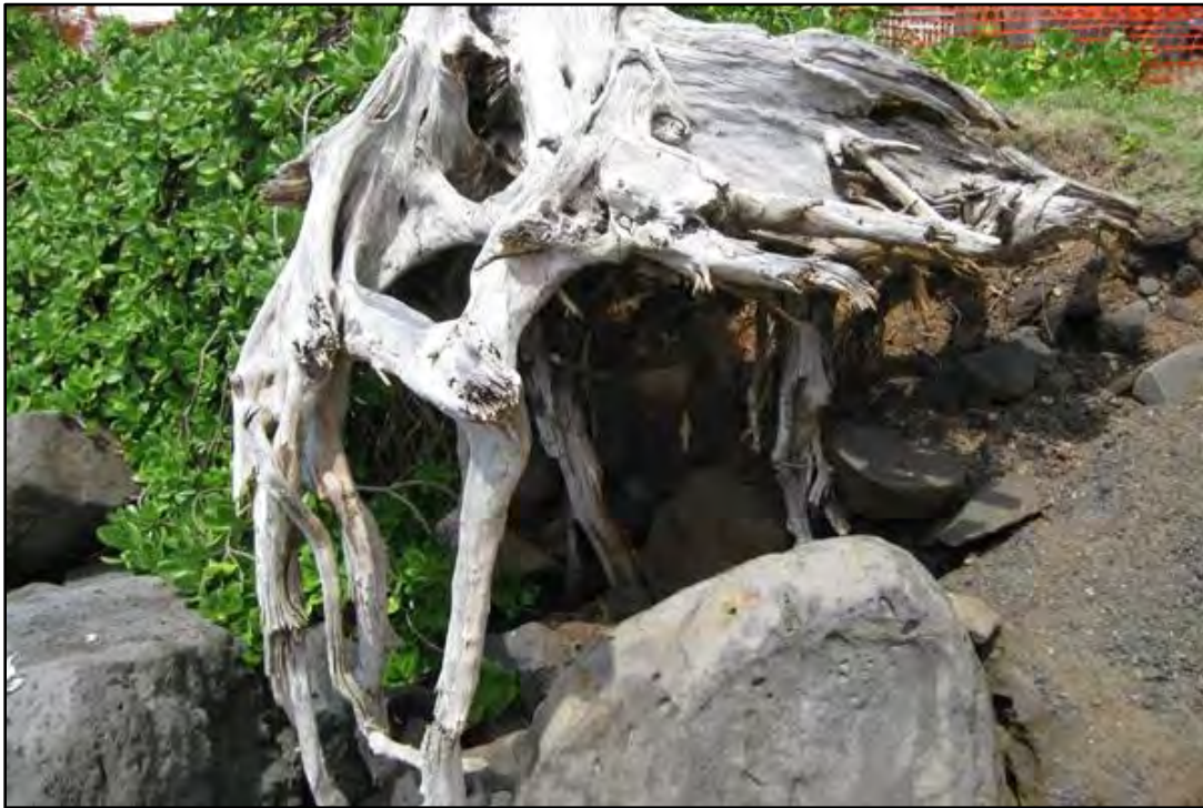
Figure 2-18 Erosion around northern stump at Station 8+40
