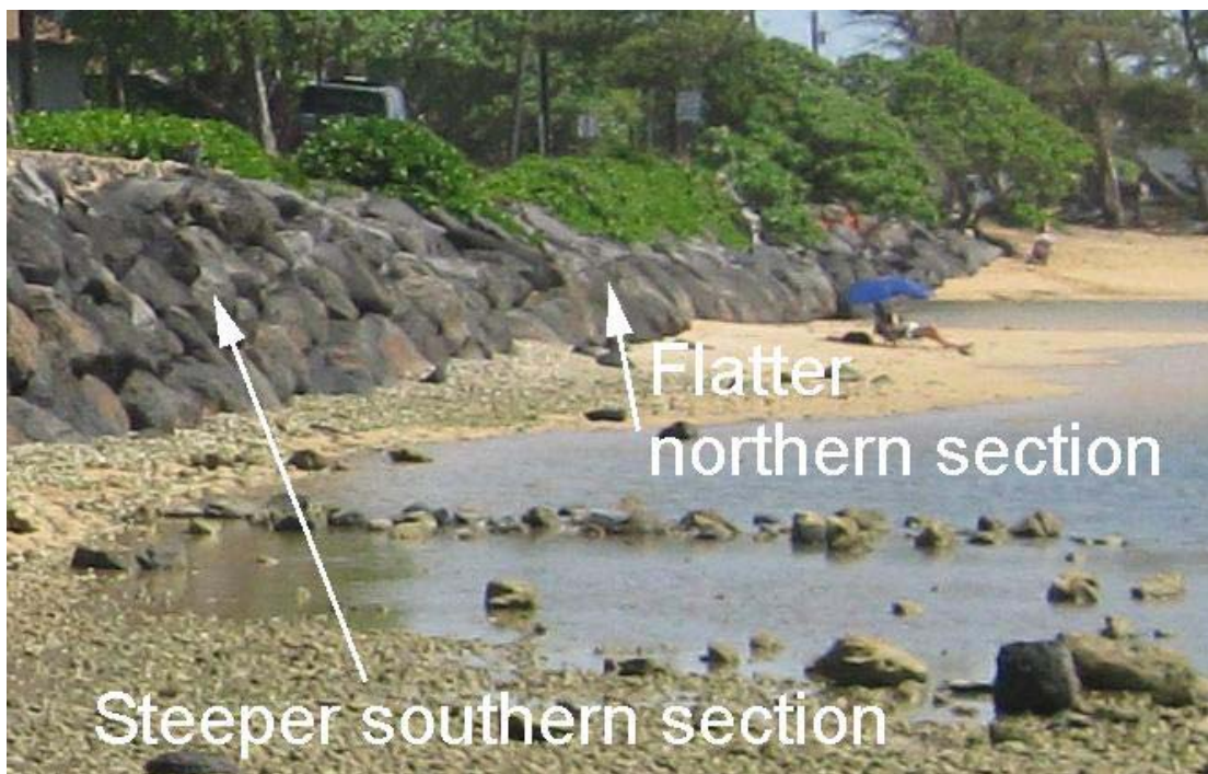
Photo 6: Transition between revetment profiles (Source: Sea Engineering, Inc.)
