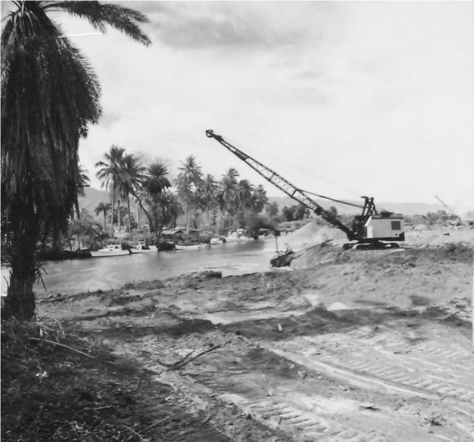
Figure 47 Construction of the Hale'iwa Boat Harbor ca. 1960
