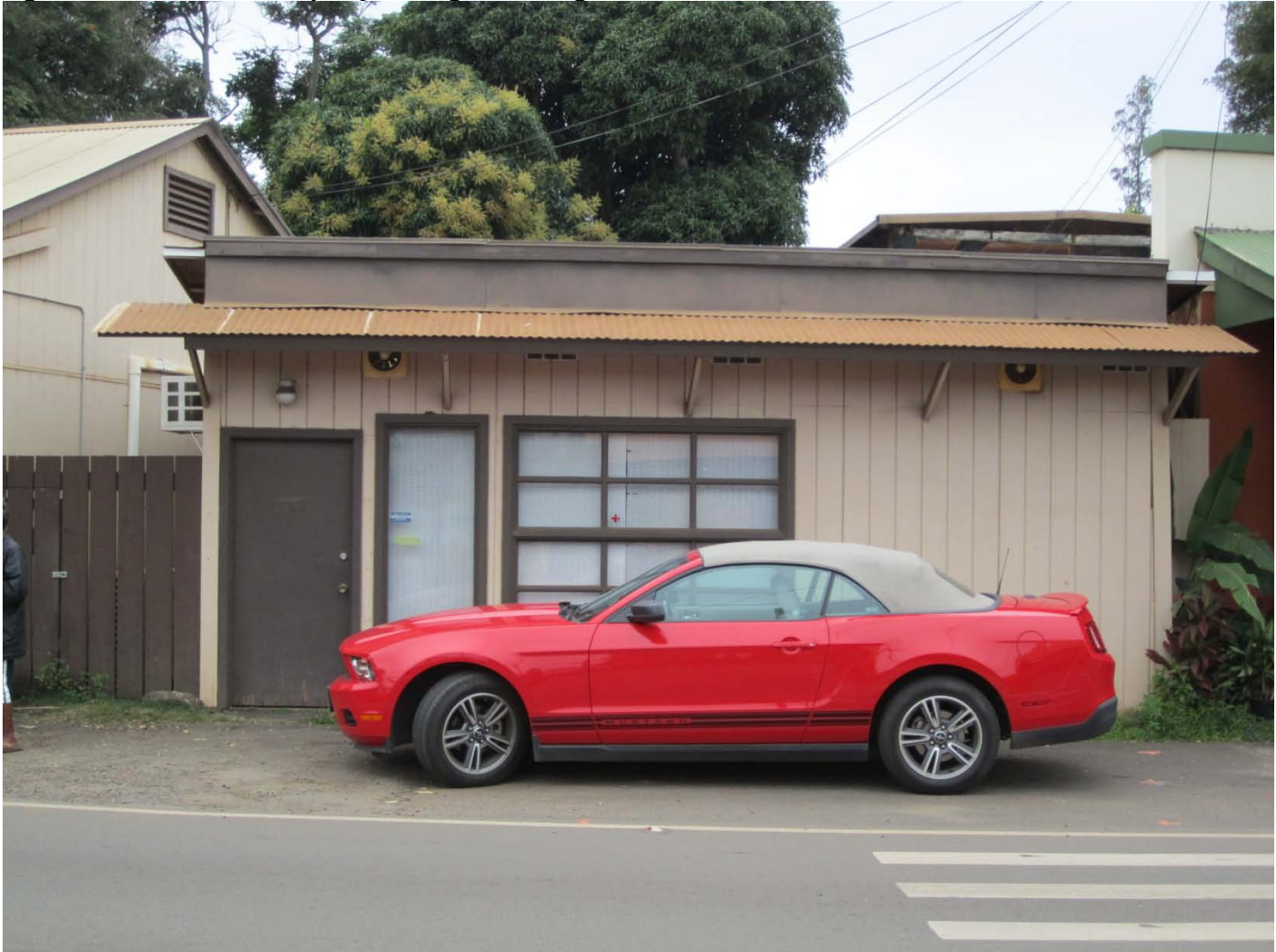
Figure 18 Matsumoto Property Storage Building 2B
