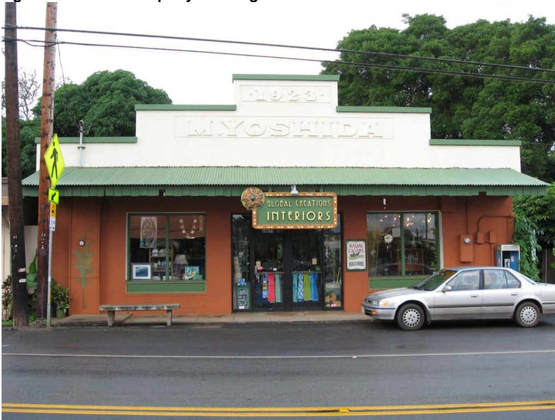
Figure 16 Yoshida Property Building 1B
