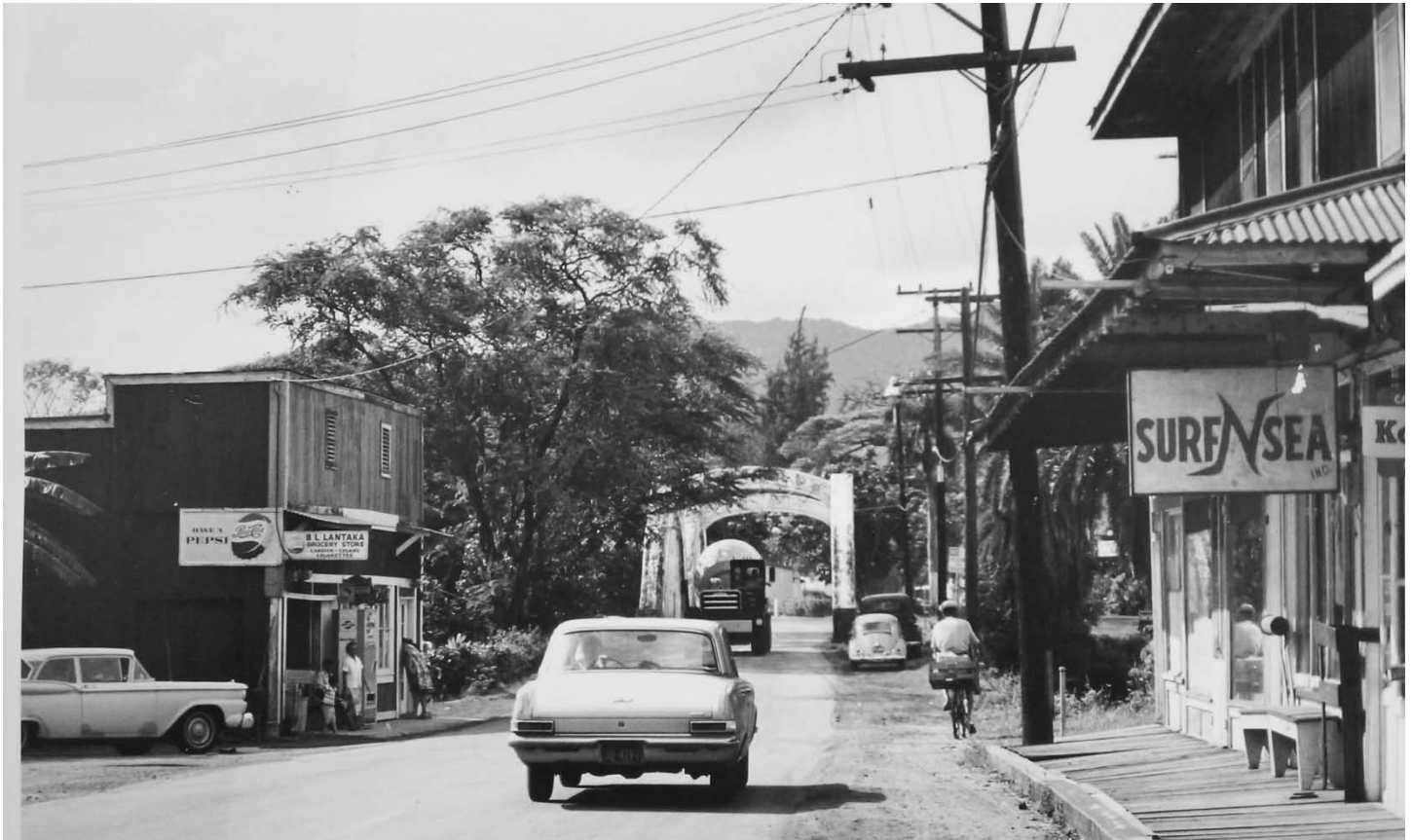
Figure 46 View from north of the Anahulu Bridge looking towards the WSL ca. 1960
