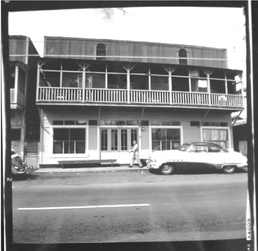
Figure 34 Two-story wood frame building along Kamehameha Highway ca. 1960
