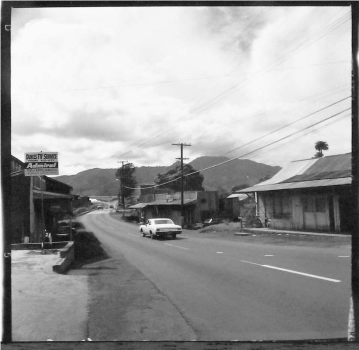
Figure 30 View from Kamehameha Highway looking South towards Weed Junction ca. 1960
