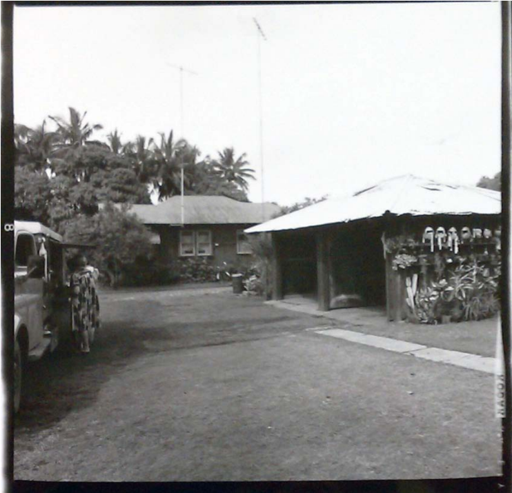
Figure 40 Housing around the WSL 1 ca. 1960
