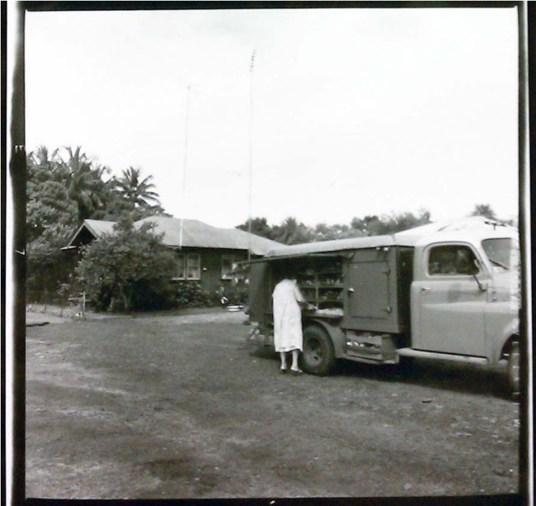
Figure 41 Housing around the WSL 2 ca. 1960
