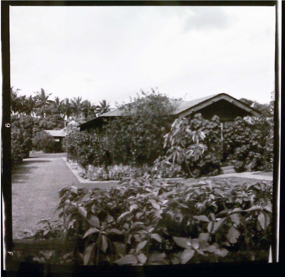
Figure 43 Housing around the WSL 4 ca. 1960
