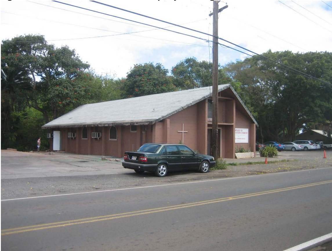
Figure 20 House of the Restoration Property Building 3
