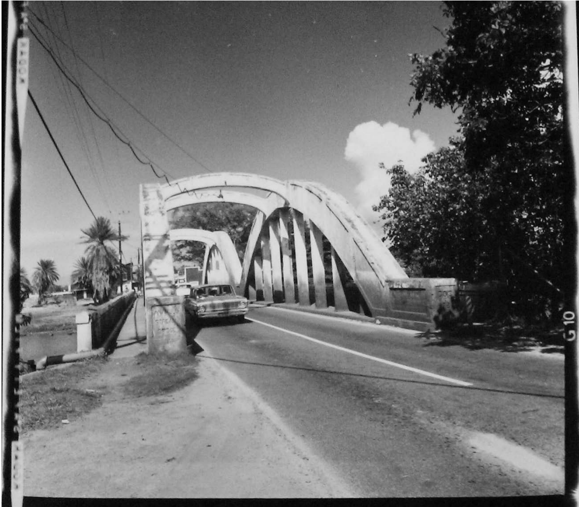
Figure 23 Anahulu Bridge looking North ca. 1960
