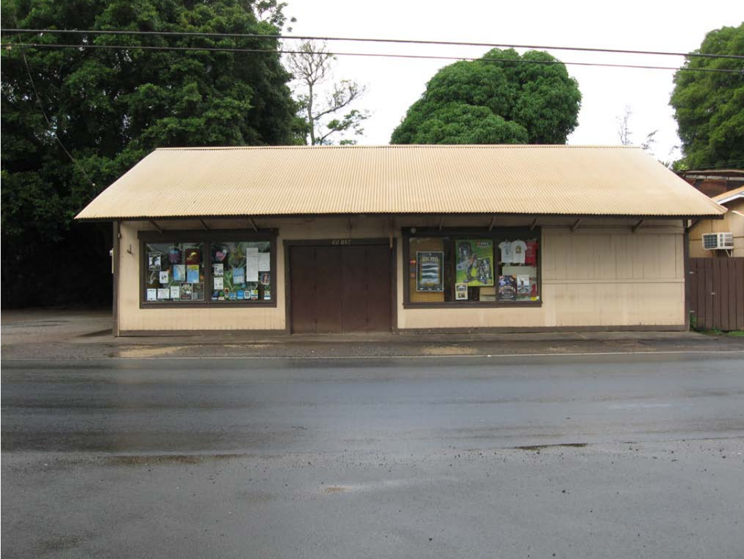
Figure 17 Matsumoto Property Store Building 2A
