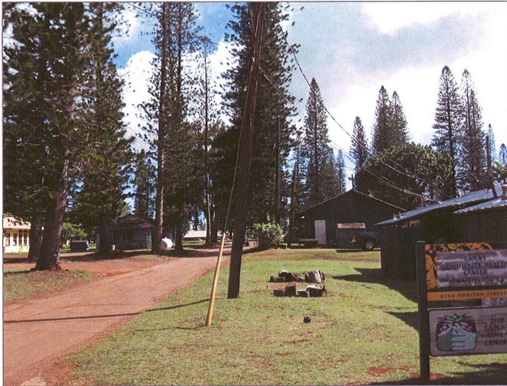
Photo1: Existing Health Center office and propane gas tank – looking east on Houston Street
