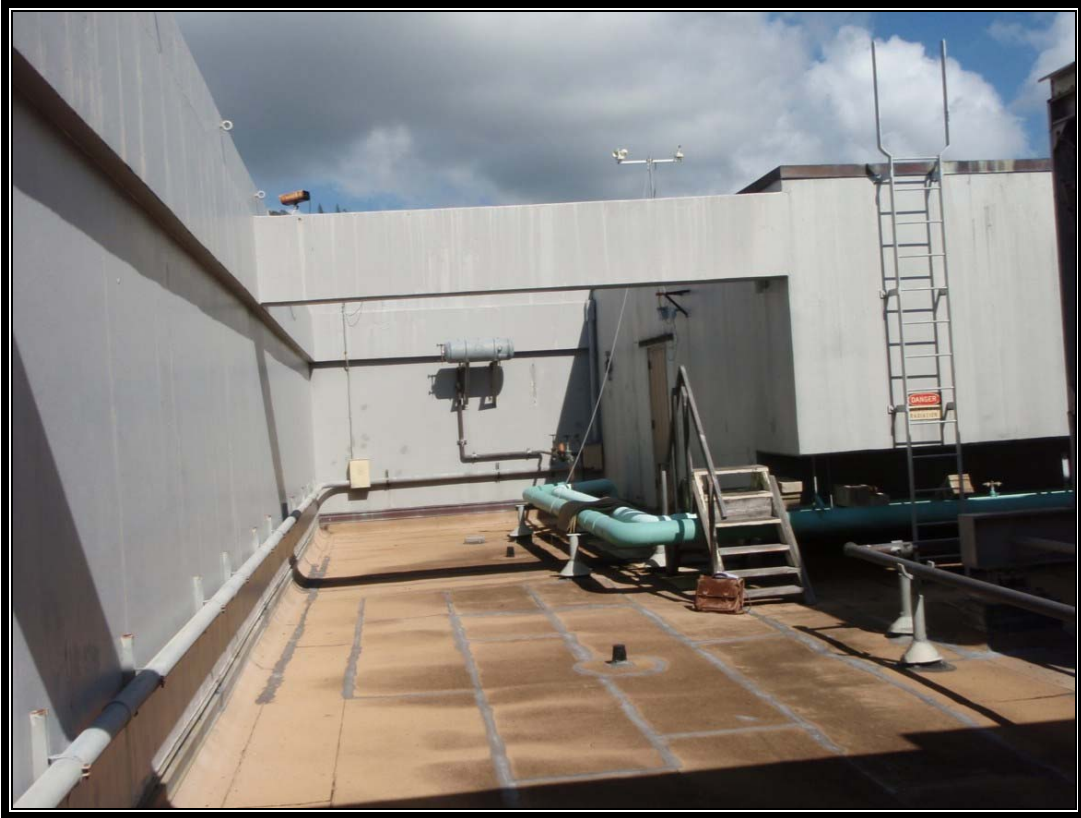
View north of roof access
