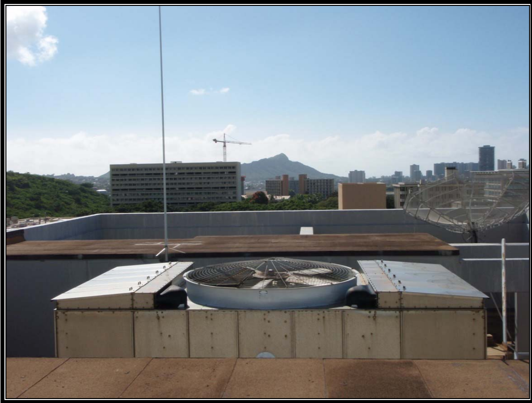
View south of roof area and Diamond Head
