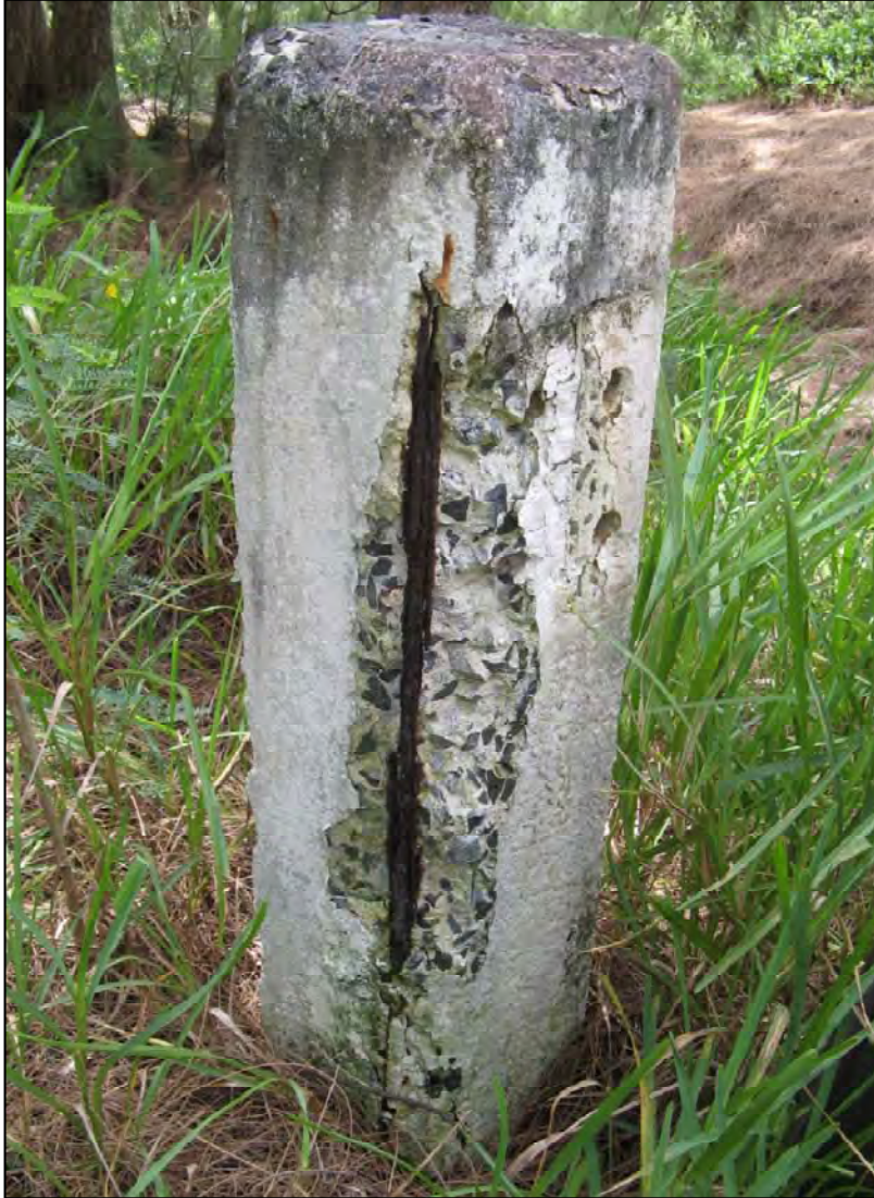
Figure 13. Concrete post showing exposed rebar. Note: the holes on the right of post were used to secure a guardrail now missing.
