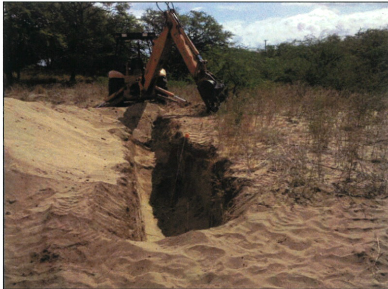
Photo # 13: BT-11 Post Excavation Overview to Northeast.
