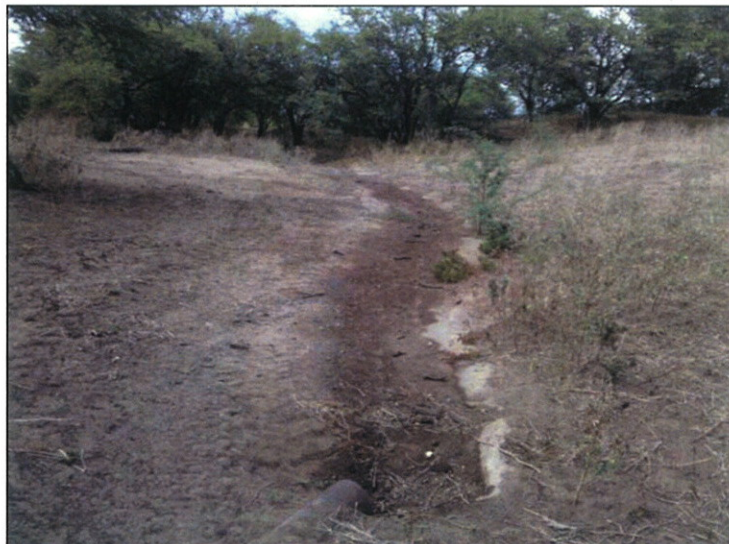
Photo # 17: Runoff draining through a small ditch (sections partially concreted), view to northeast.
