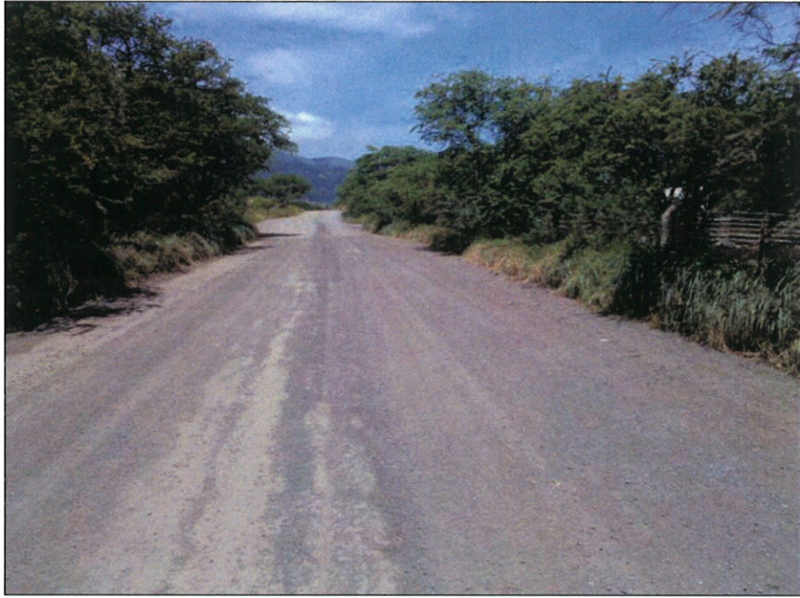
Photo # 4: Graded Access Road Bisecting the Western Portion of the Project Area, View to Northwest.
