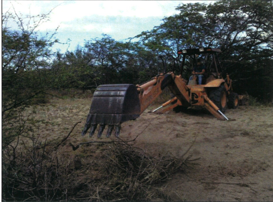
Photo # 7: Overview of BT-5 Excavation (sandy surface), view to northwest.
