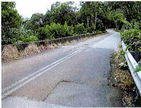
Figures 17 and 18: "Hogsback", near Mile Marker 4.0 Basalt (lava rock) retaining wall at Hogsback.
