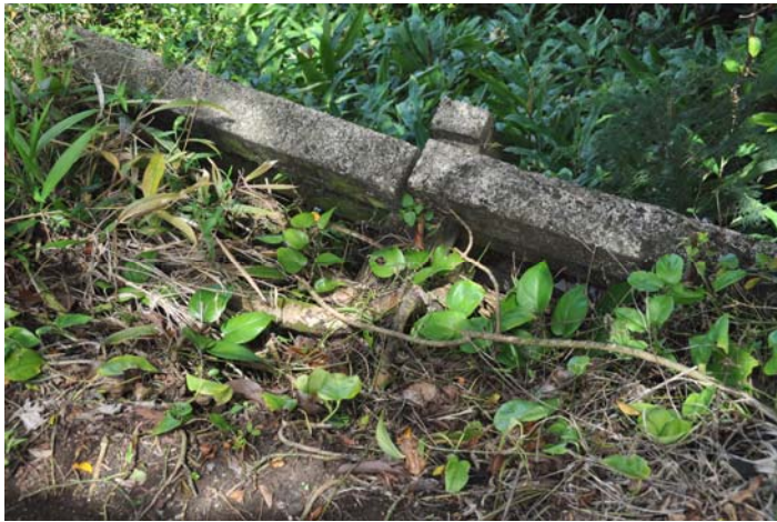
Photo 4. Top of crib wall structure, adjacent to roadway
