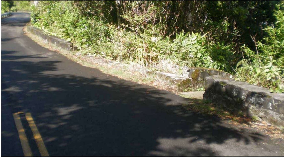
Figure 16. Photograph showing the culvert at the southern end of the low basalt and concrete guard wall along the southwestern (Pauoa Valley) side of Tantalus Drive, view to west. Note that the guard wall continues south of the project area along the ‘Hogsback.’
