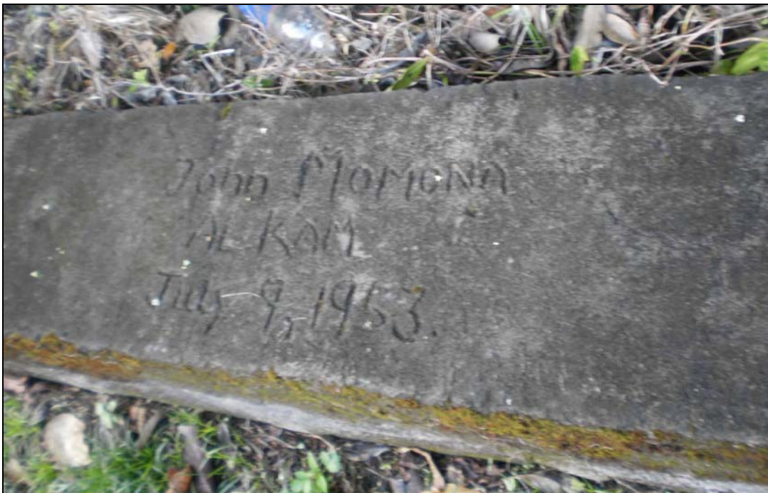
Figure 15. Photograph showing the inscription (John MOMONA AL KAM July 9, 1953) on the top of the southern end of the low basalt and concrete curb along the southeastern (Makiki Valley) side of Tantalus Drive
